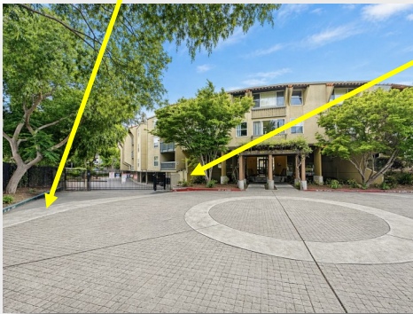
LOCKBOX STATION IS TO THE RIGHT OF THE MAIN GATE.
