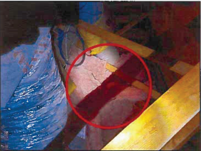
Insulation has been moved
