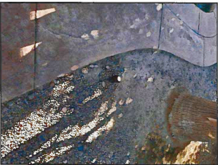
Lights work on timer
