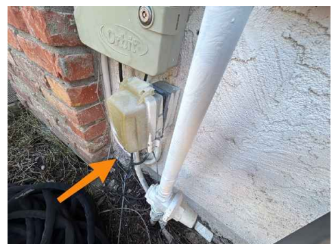
Front of Property
