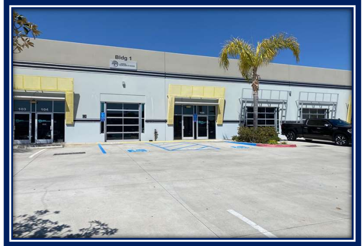
View of subject units from parking area.
