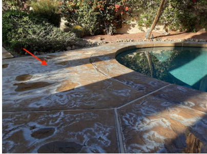
Hard Water Buildup
