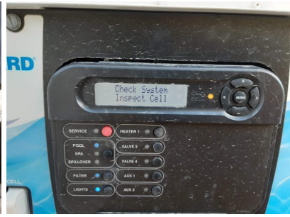
Check System - Inspect Cell
