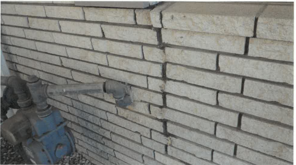
Grout damage and cracked brick fascia
