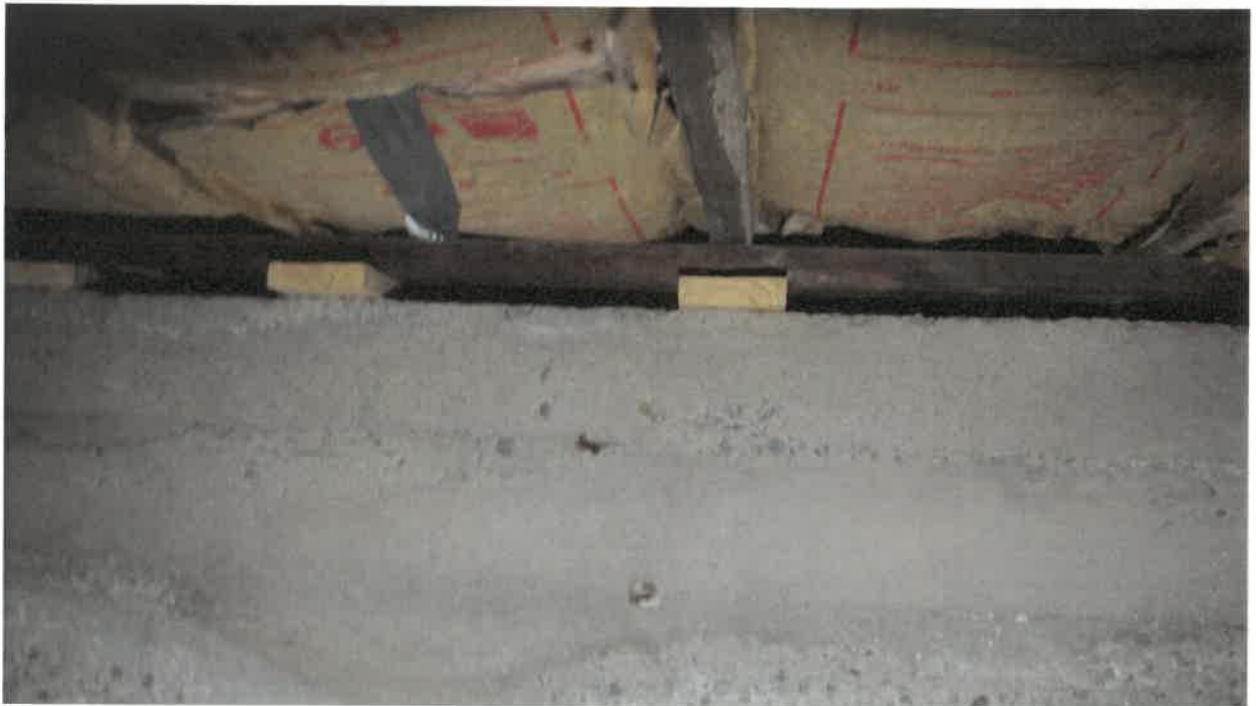
Wood shims at sill plate to foundation wall connection
