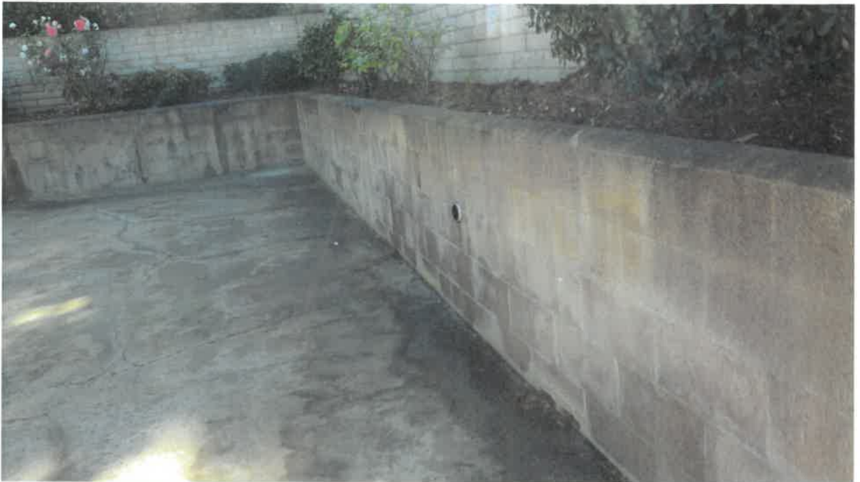
Water damaged site retaining walls
