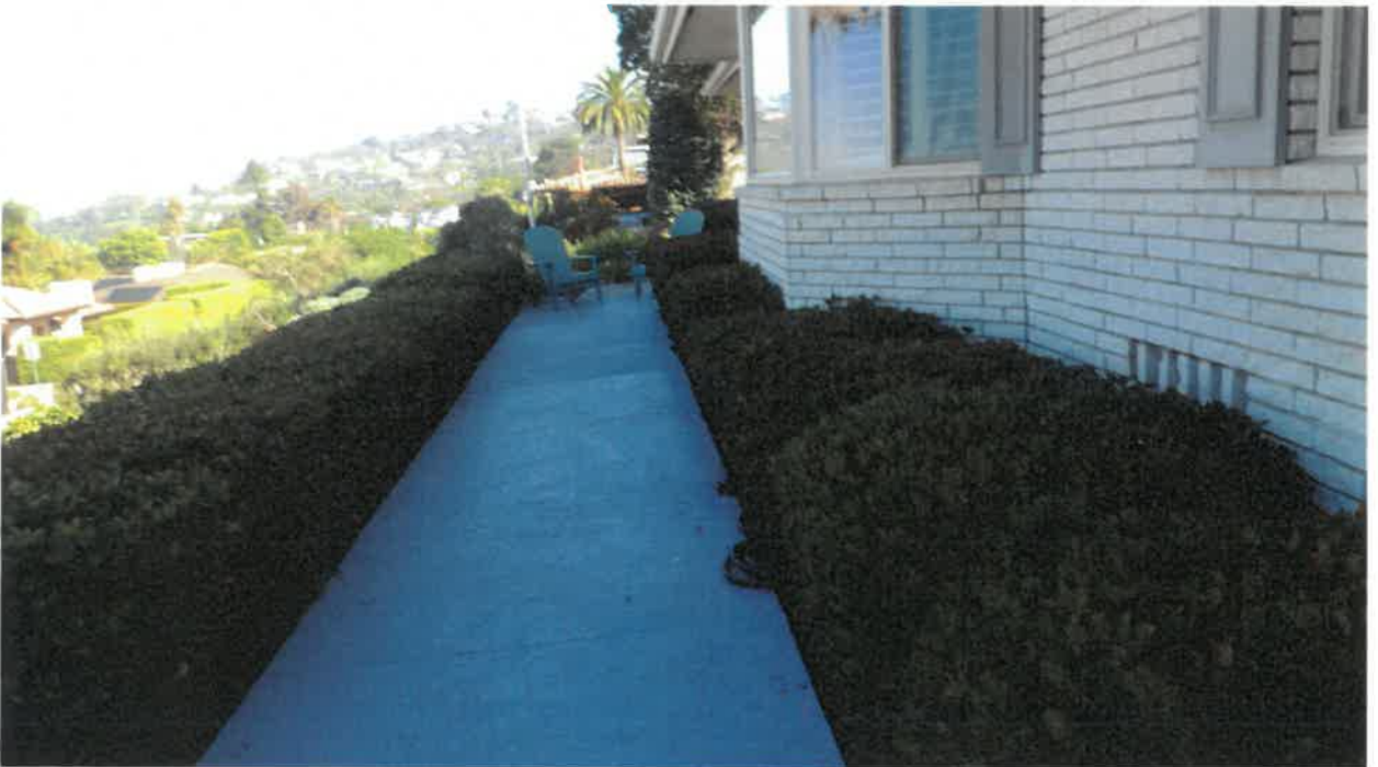
Confined planter with vegetation and irrigation adjacent to south foundation wall
