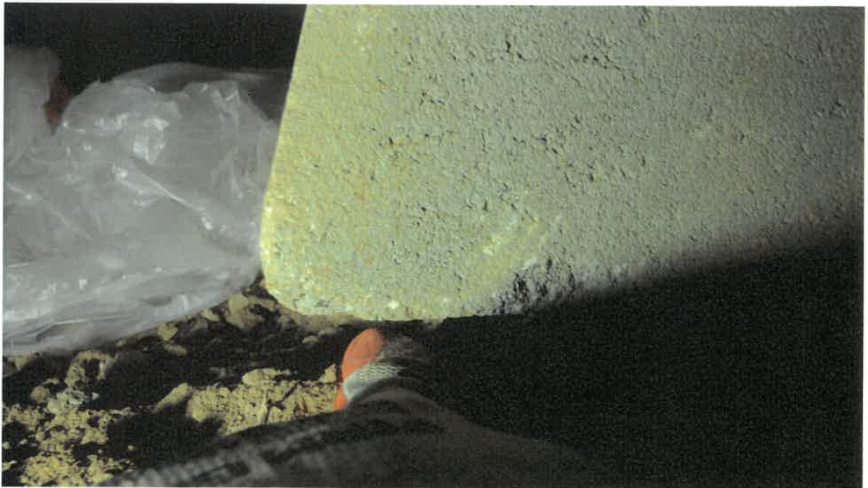
Modern precast footing with no embedment
