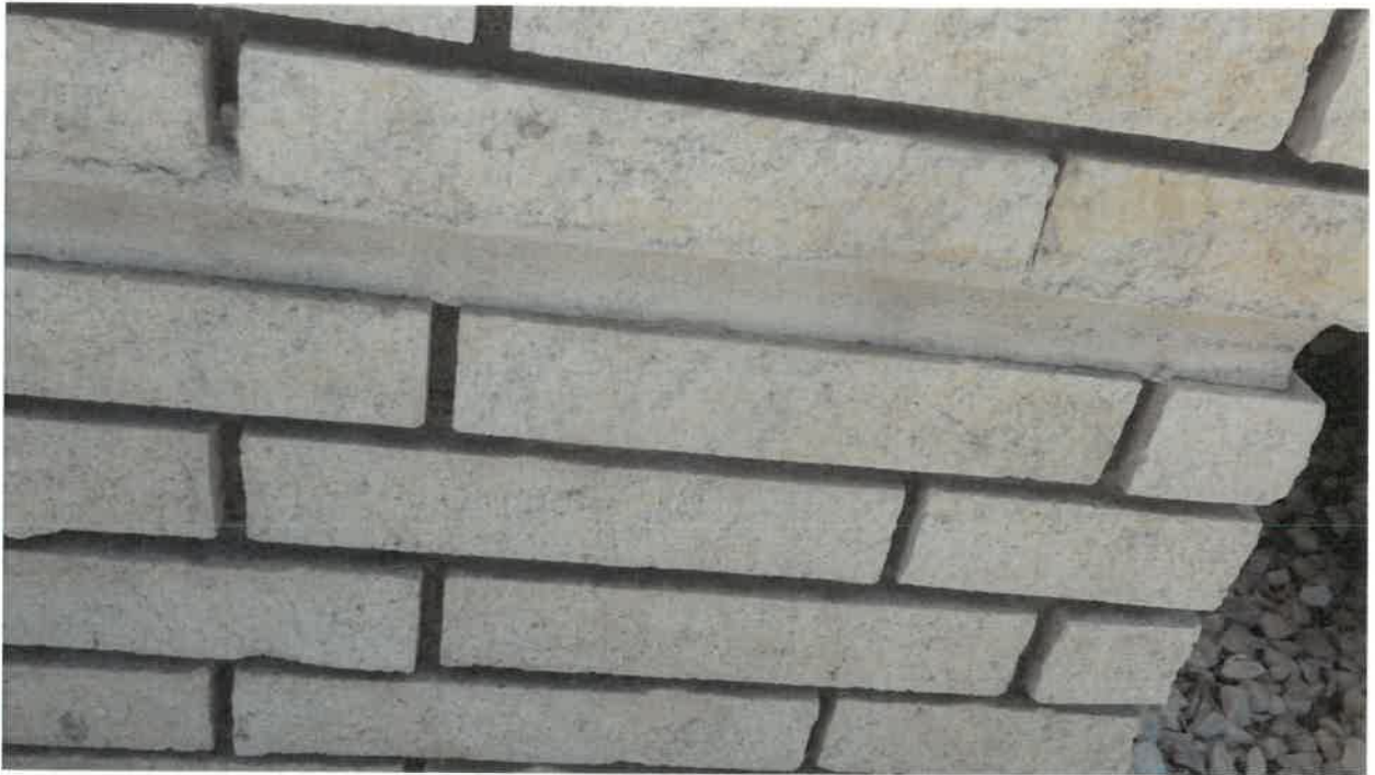
Large grout along south brick fascia
