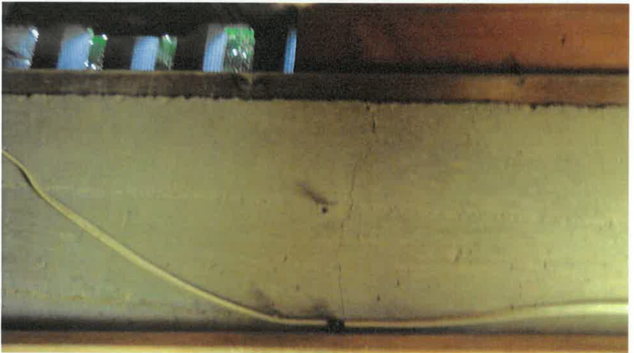
Foundation wall cracks
