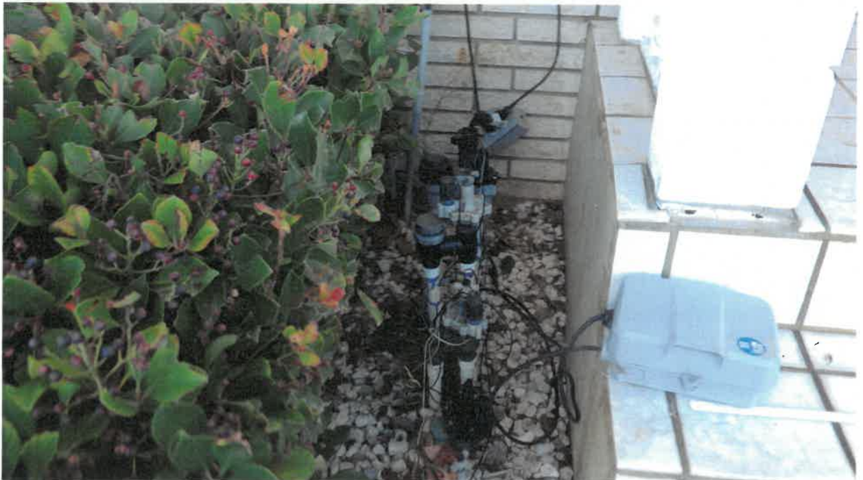
Irrigation manifold adjacent to residence
