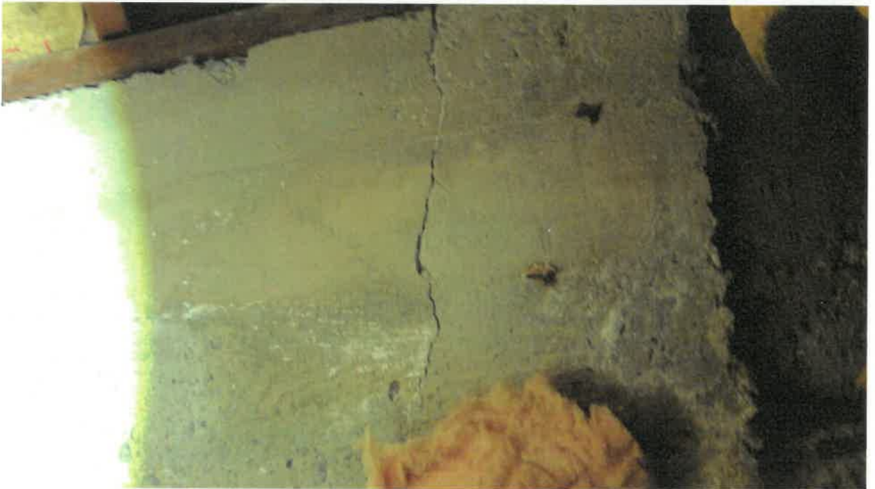
Foundation wall cracks
