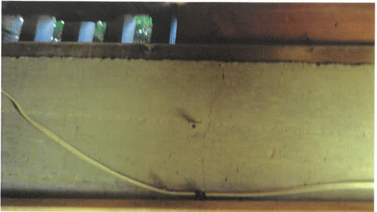
Foundation wall cracks
