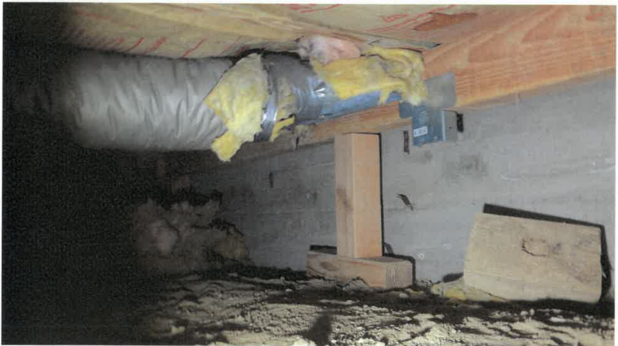
Wood post and beam supported by wood block along south foundation wall
