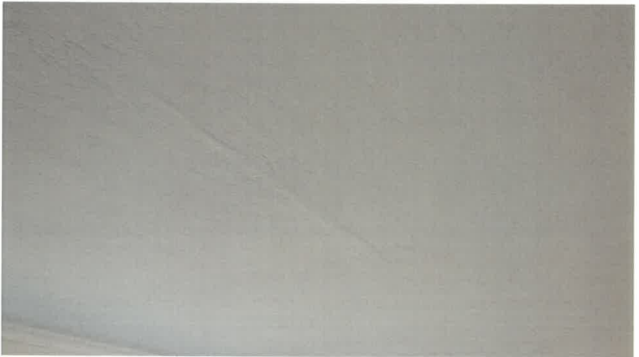
Plaster cracks
