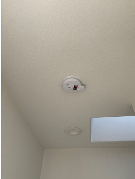
2nd Floor Hallway
