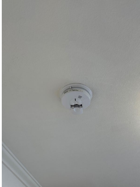
1st Floor Hallway
