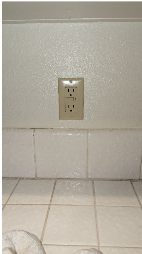
Kitchen and both Bathrooms replaced with GFCI outlets.
