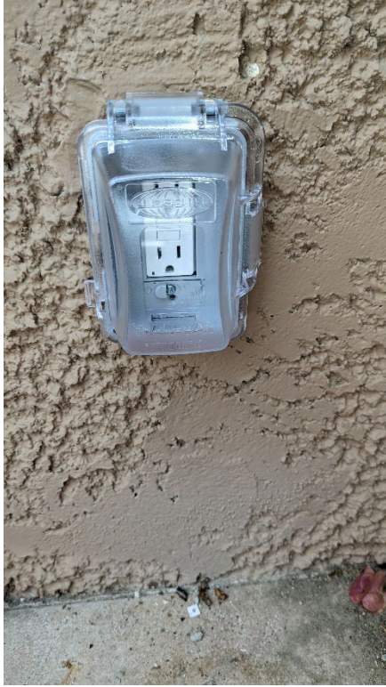
Garage outlet replaced with GFCI. And the polarity issue resolved.
