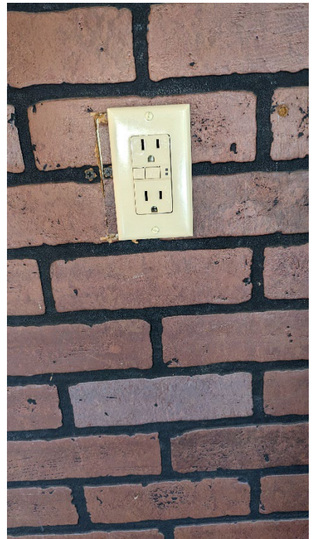
Garage outlet replaced with GFCI. And the polarity issue resolved.
