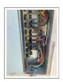
**4.2** Conductors are clearly marked. Grounded conductors are marked white or gray and equipment grounding conductors (EGC) shall be green, green/yellow, or bare. NEC 200.6, 250.119, 310.110: Yes. All to code.
