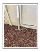
**4.4** Conduit rated for location with supports properly spaced for size and type of conduit NEC 358, NEC 352, 350.22: All conduit is underground with this installation method.
