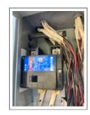
2.2 Primary PV Breaker Size: 1 breaker at 30 Amps.
