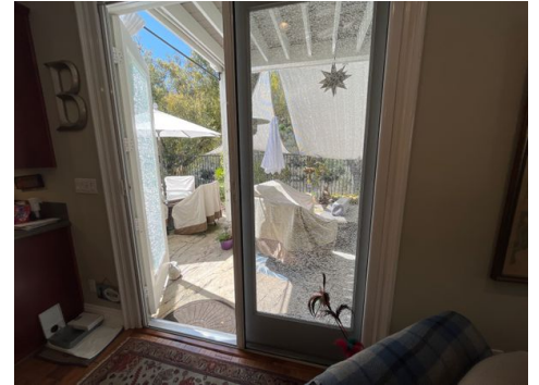
Example Noted at Kitchen
