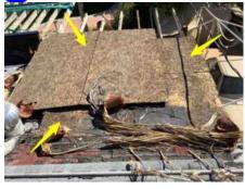
NR Improper installation at patio roof.
