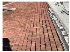
NR Damaged or missing Shingles noted. Repair/Replacement needed.
