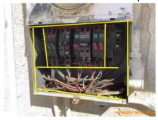
The main electrical service panel was made by Zinsco. Zinsco panels are reputed to have a high rate of circuit breaker failure which can result in a fire or shock/electrocution. The Inspector recommends that before the expiration of your Inspection Objection Deadline, you consult a qualified Electrical Contractor to have panel inspected for any issues and possible replacement. Information about defective Zinsco panels is widely available on the internet.
