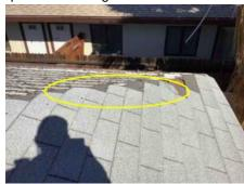
NR Debris should be removed from roof, Recommend further review and repair by a qualified Roofing Contractor
