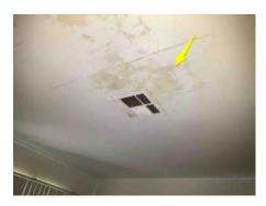
Stains noted to ceiling in rear room, roof appears to be leaking. We recommend further review and repairs by a qualified specialist in the appropriate trade.
