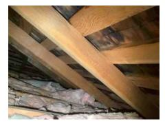
RM Uneven insulation noted, recommend adding addition insulation.
