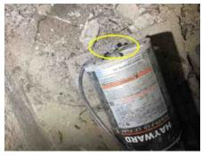
If wire to pool shell can not be found. Contact a qualified Pool Contractor about installing a water bond system.
