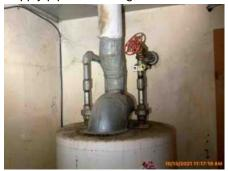
NR Shut off valve at water heater is seized, We recommend the advice and services of a State Licensed Plumbing Contractor
