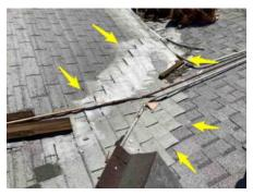
Heavy Wear noted to composition roof, composition roof appears to be at its end of its service life. Recommend the entire roof be evaluated and repaired by a qualified Roofing Contractor.
