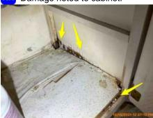
Moisture damage and mold like substance noted at cabinet under sink. We recommend further review and repairs by a qualified specialist in the appropriate trade.
