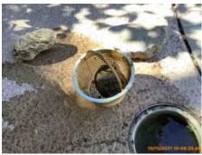
BM Debris in skimmer, cleaning is needed. Weekly cleaning is recommended.
