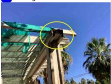
Moisture damage noted to front porch roof sheathing, Recommend further evaluation by a qualified Termite Company
