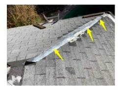
NR Repairs appear to be substandard. Recommend the entire roof be evaluated and repaired by a qualified Roofing Contractor
