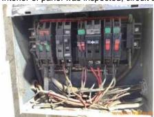
Multiple wires are connected to a single lug on a circuit breaker where only one wire should be connected. Recommend further review and repair by qualified Electrical Contractor.
