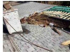
Nails/Fasteners are protruding from the roof surface. Recommend the entire roof be evaluated and repaired by a qualified Roofing Contractor\_\_\_\_
