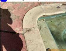
The deck has cracked and lifted causing a trip hazard, We recommend further review and repairs by a qualified specialist in the appropriate trade.
