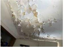
Ceiling panels separating, damaged and missing in rear room. We recommend further review and repairs by a qualified specialist in the appropriate trade.
