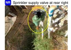
NR Sprinkler main supply line shut off valve handle leaking at front
