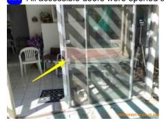
Glass tempered markings are not visible at some exterior doors, replacement should be considered to all non tempered sliding doors and fixed windows. Fed law requires companies to replace none tempered glass doors. They are not allowed to repair them.
