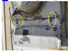
Dead front cover missing at main electrical panel, this is a safety concern, installation is needed for safety, Recommend further review and repair by qualified Electrical Contractor.
