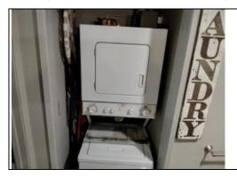
**Advisory:** Rubber Hoses are installed on the washing machine. Rubber laundry hoses are susceptible to fail without warning. Recommend installing braided metal hoses when the hoses are replaced.
