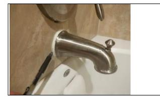
**Repair:** The tub/shower diverter was found to be difficult to operate or was not fully operative in the bath. We recommend repair or replacement of the diverter(s).
