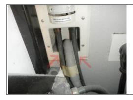
Advisory: The laundry vent discharge is above the vent on the dryer. This means that the lint must be blown uphill before it is discharged. Most dryer lint motors are too small to efficiently remove the lint from the hose. Recommend that the vent hose be cleaned annually to reduce the possibility of fire originating in the hose.
