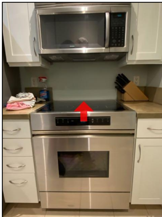
30. Backsplash/heat shield recommended
