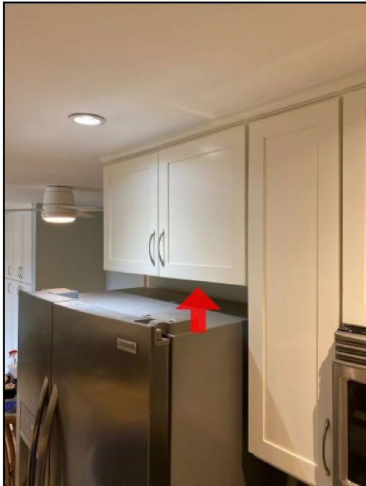
28. Cabinet doors/drawers - Adjustment needed
