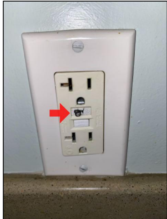
14. Damaged outlet
