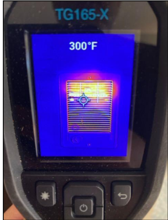
17. Functional at the time of the inspection
