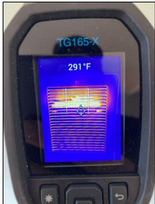
19. Functional at the time of the inspection
