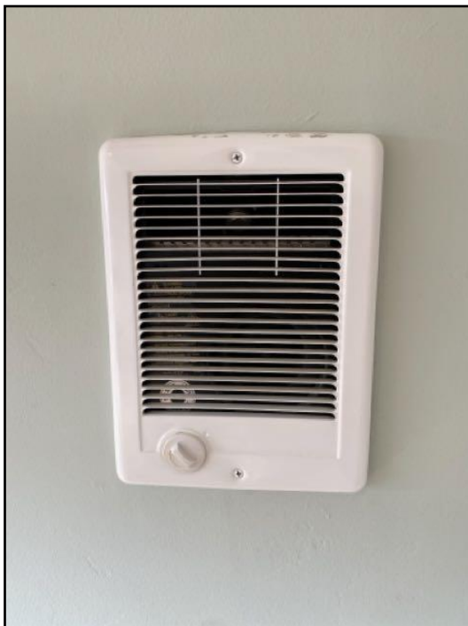
18. Electric wall mounted heater(s)...
