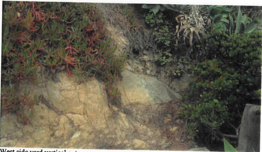
West side yard vertical cut
