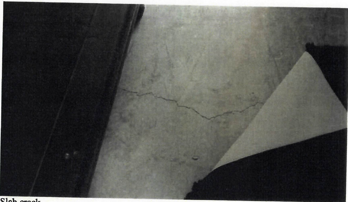
Slab crack
