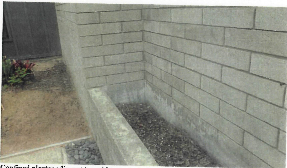
Confined planter adjacent to residence
