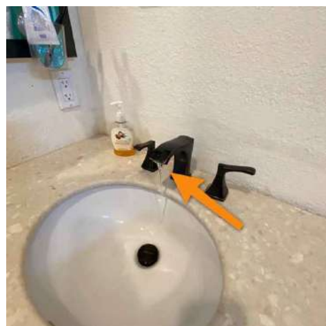
Upper Hall Bathroom
