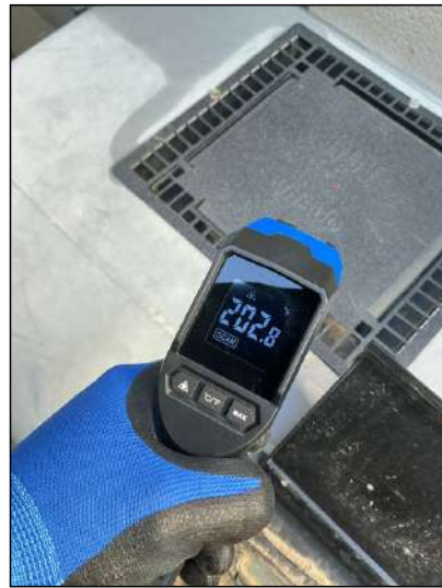
Thermal thermometer reading on heater exhaust: 202 degrees
