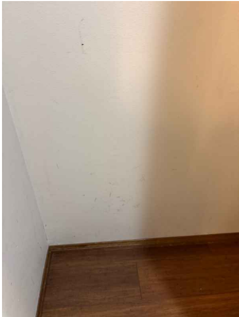
Example Primary Bathroom
