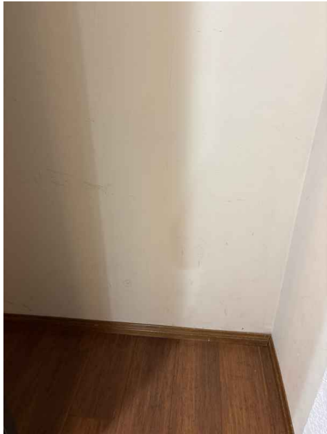
Example Primary Bathroom
