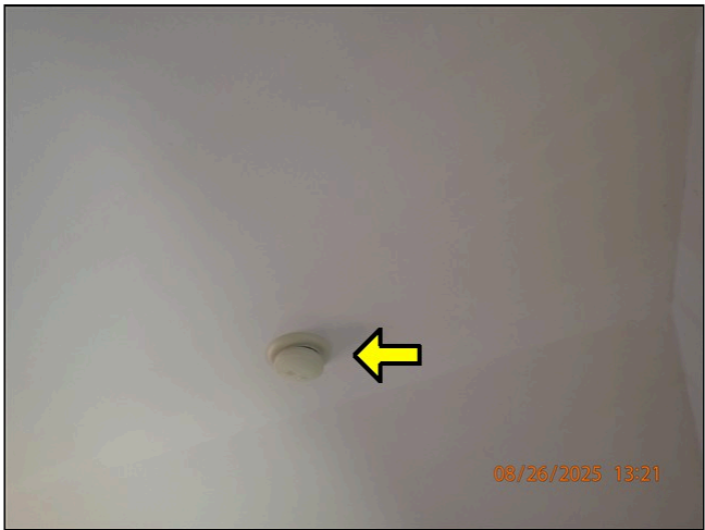
10.0 Item 1 (Picture) (2) Photo of a smoke detector(s).
