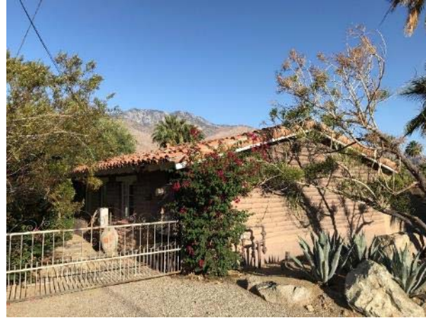
2275 S. Araby Dr., view west/northwest showing adobe construction. ARG, 2021.
