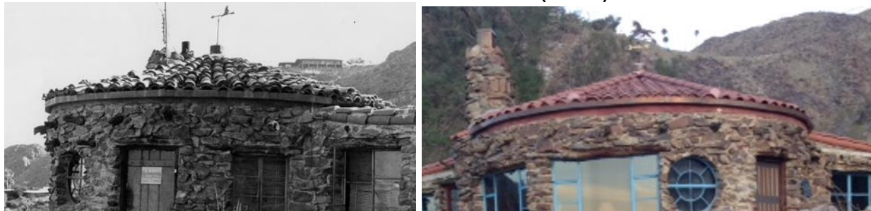
BELOW A COMPARISON OF THE ORIGINAL CLAY TILE ROOF (c. 1953) AND REPLACEMENT ROOF.
