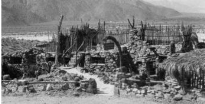
BELOW AN EARLY VIEW, SOUTH FAÇADE OF 2550 S. ARABY
