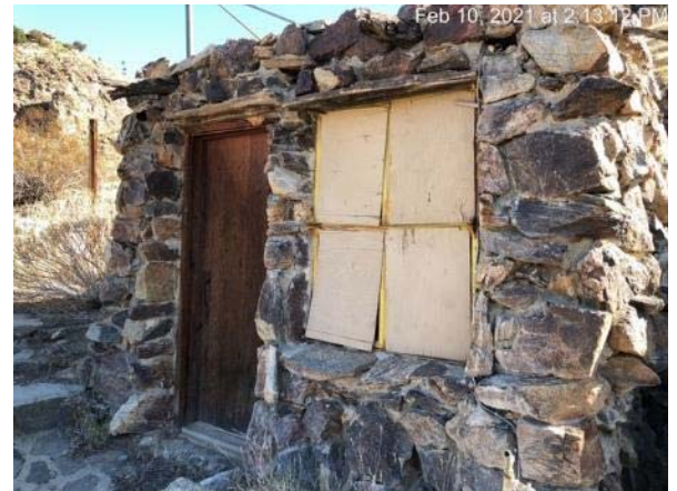
2500 S. Araby Dr., entry detail, view south. City of Palm Springs, 2021.
