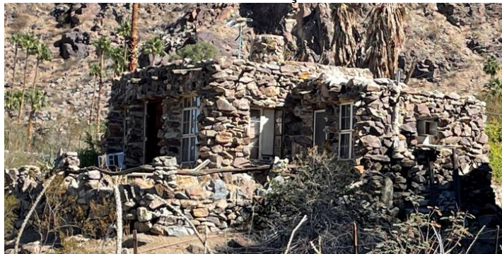
BELOW RECENT VIEW WEST FAÇADE OF 2550 S. ARABY
