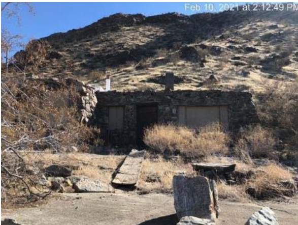
2500 S. Araby Dr., primary façade, view south. City of Palm Springs, 2021.
