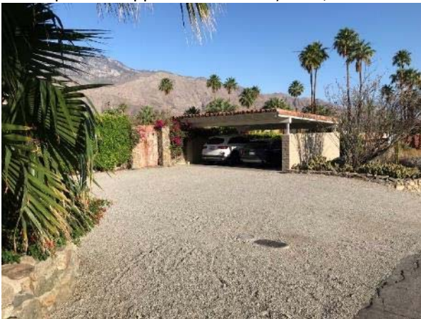
2275 S. Araby Dr. modern carport, view northwest. ARG, 2021.
