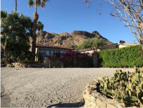
2275 S. Araby Dr. overview, view southwest (all visible portions appear to be adobe). ARG, 2021.
