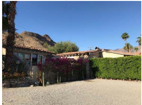
2275 S. Araby Dr., view southwest (all visible portions appear to be adobe). ARG, 2021.
