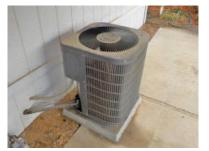
Fuel Source: No electrical disconnect in line of site / next to
