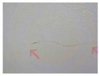
Master Bath: There is some minor cracking in the sheetrock. Most likely this is due to slight
