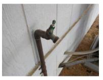
The temperature pressure relief valve at the upper portion of the water heater is a required safety valve which should be connected to a drain line of proper size terminating just above floor elevation. If no drain is located in the floor a catch pan should be installed with a drain extending to a safe location. The steam caused by a blow-off can cause scalding. Improper installations should be corrected.
