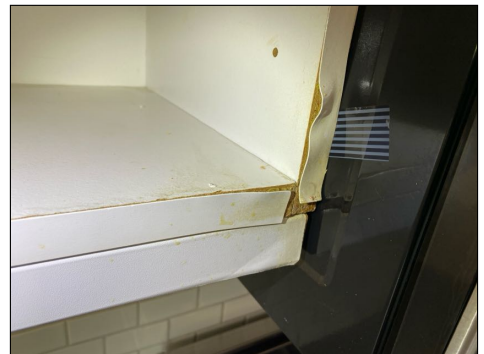
Delamination occurring in multiple areas – service needed
