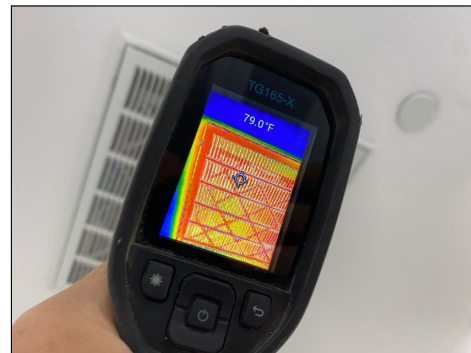
Temperature at Air Return
