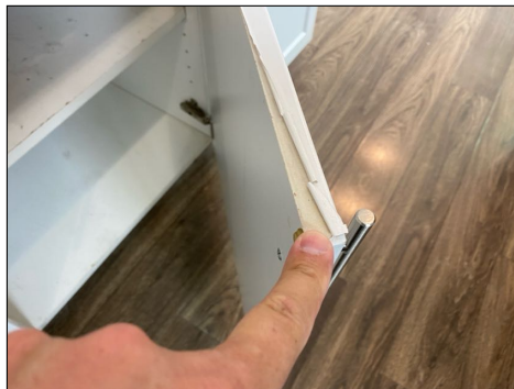
Delamination occurring in multiple areas – service needed
