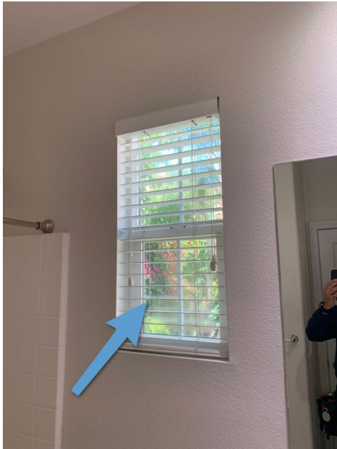
Example Noted at Shared Bathroom
