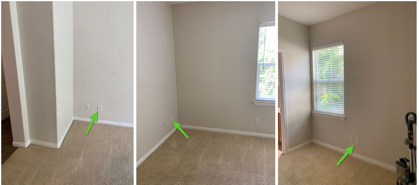
Example Noted at Master Bedroom
