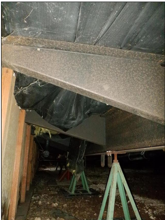
6.0 Item 7(Picture) Crawlspace
