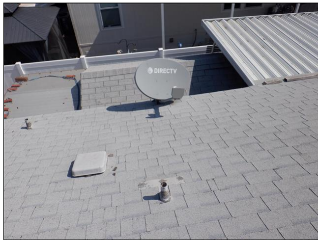
1.0 Item 6(Picture) Roof covering
