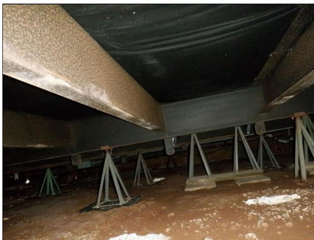
6.0 Item 10(Picture) Crawlspace
