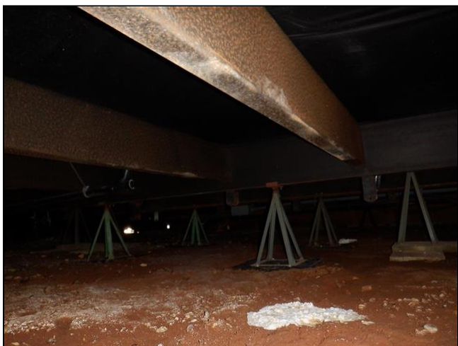
6.0 Item 9(Picture) Crawlspace
