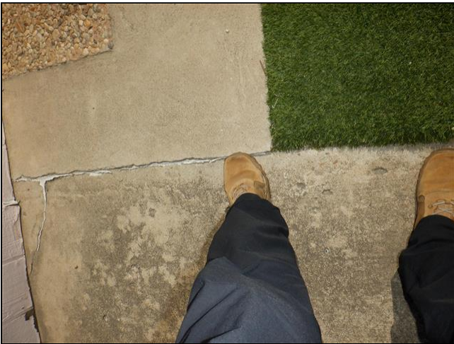
2.4 Item 1(Picture) Lifting in walkway
