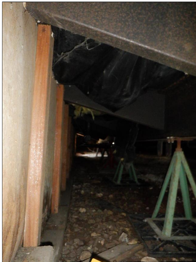
6.0 Item 6(Picture) Crawlspace
