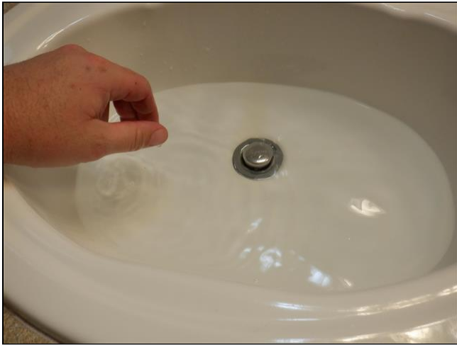
5.6 Item 3(Picture) Primary bath sink drains slowly
