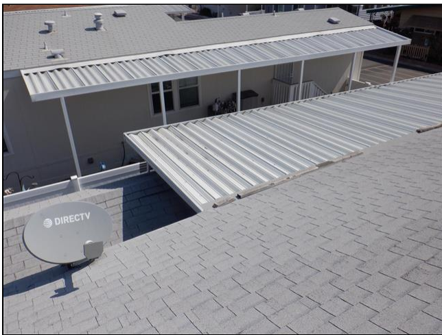
1.0 Item 5(Picture) Roof covering
