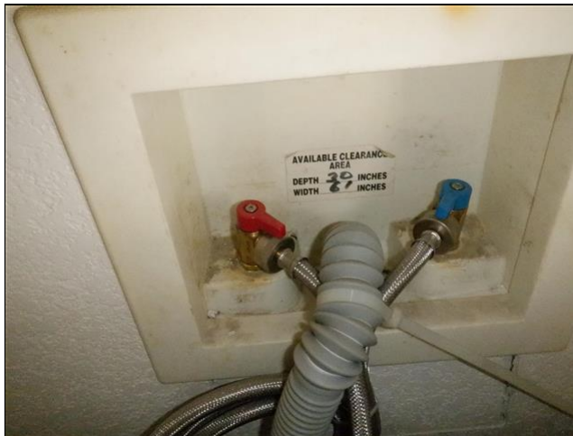
3.13 Item 2(Picture) Washer valves / drain
