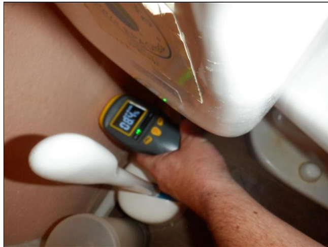
5.1 Item 2(Picture) Moisture test around hallway bath plumbing
