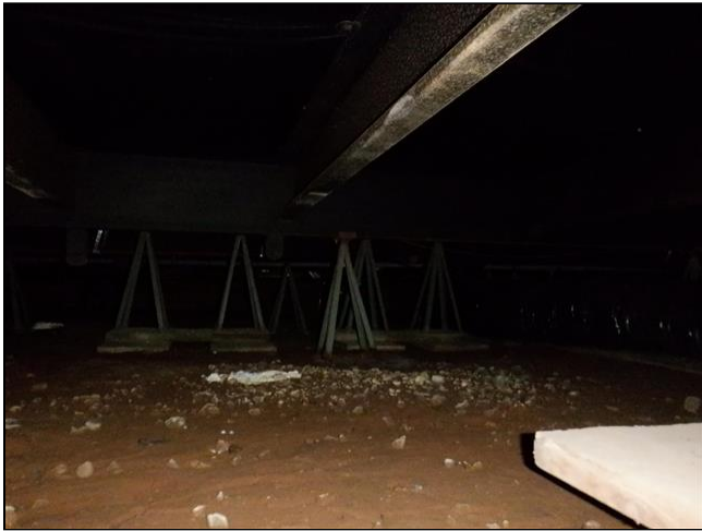
6.0 Item 11(Picture) Crawlspace
