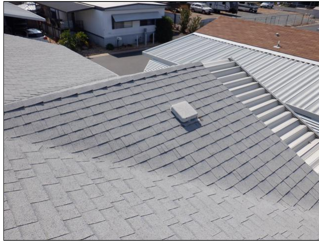
1.0 Item 8(Picture) Roof covering
