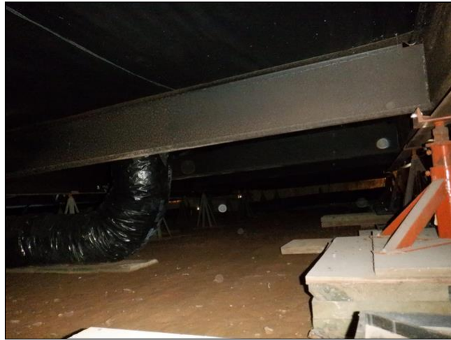
6.0 Item 12(Picture) Crawlspace
