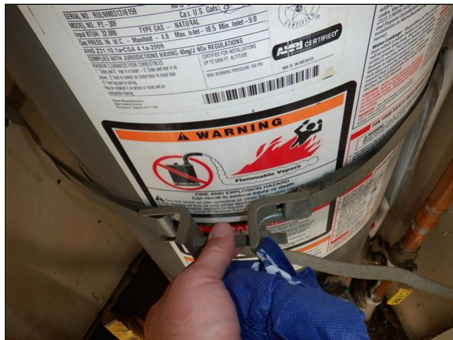
7.1 Item 4(Picture) Loose belly straps
