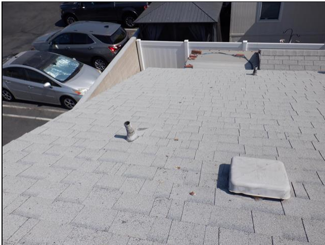
1.0 Item 1(Picture) Roof covering
