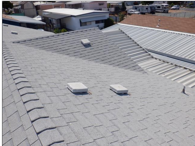
1.0 Item 2(Picture) Roof covering
