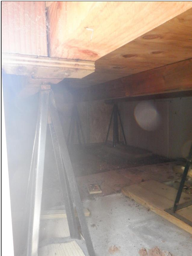
6.2 Item 1(Picture) Steel jacks under deck
