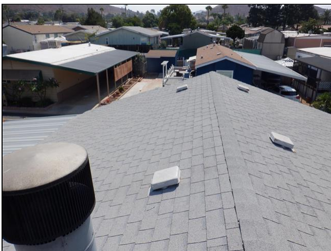
1.0 Item 9(Picture) Roof covering
