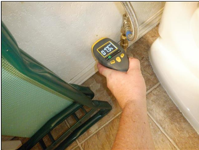
5.1 Item 1(Picture) Moisture test around primary bath plumbing
