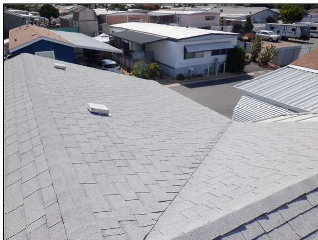
1.0 Item 10(Picture) Roof covering
