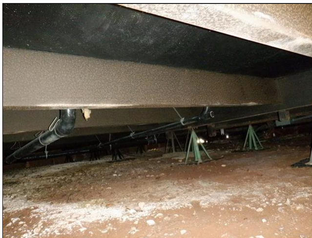
6.0 Item 8(Picture) Crawlspace
