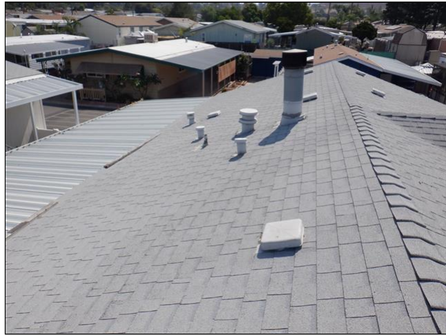
1.0 Item 4(Picture) Roof covering
