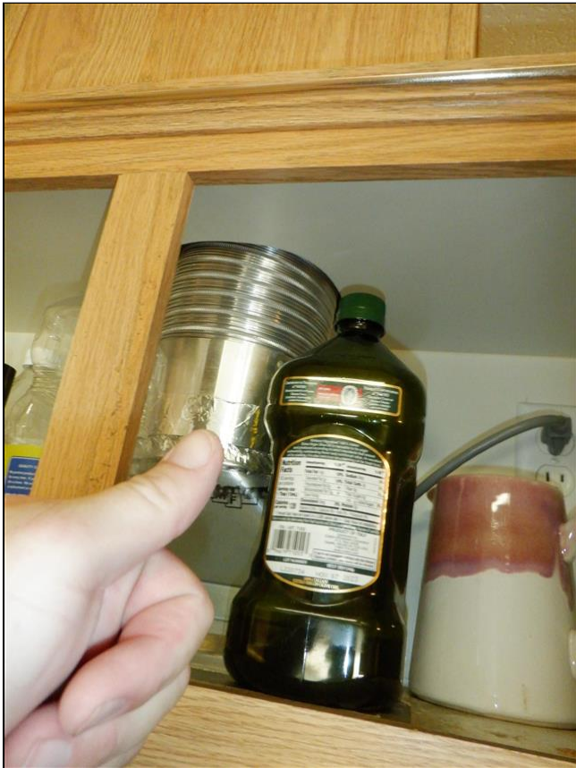
3.10 Item 1(Picture) Vent fan worked
