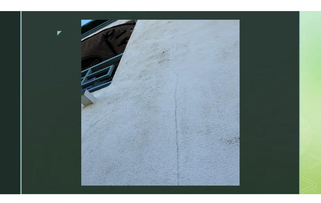
Water is getting behind the stucco and finding its way out of the top of the door assembly. Water is damaging the door assembly.
