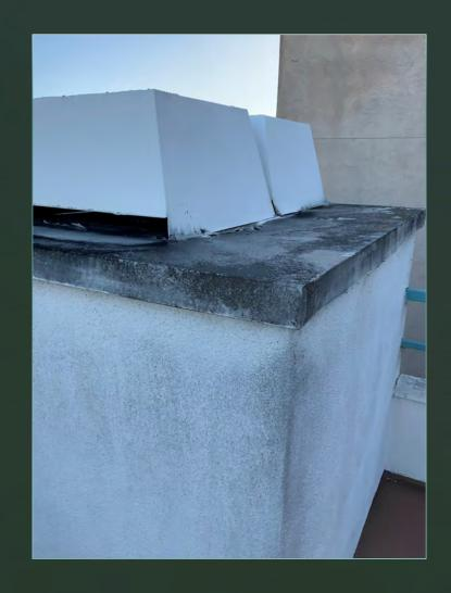
Metal Coping penetrations not sealed properly at guardrail connections. This is causing the stucco at the pony walls to bubble and crack throughout.
