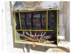
83: The main electrical service panel was made by Zinsco. Zinsco panels are reputed to have a high rate of circuit breaker failure which can result in a fire or shock/electrocution. The Inspector recommends that before the expiration of your Inspection Objection Deadline, you consult a qualified Electrical Contractor to have panel inspected for any issues and possible replacement. Information about defective Zinsco panels is widely available on the internet.
