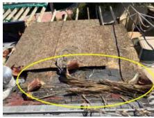
NR 18: Improper installation is found, Recommend the entire roof be evaluated and repaired by a qualified Roofing Contractor
