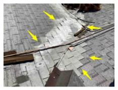
**20:** Heavy Wear noted to composition roof, composition roof appears to be at its end of its service life. Recommend the entire roof be evaluated and repaired by a qualified Roofing Contractor.
