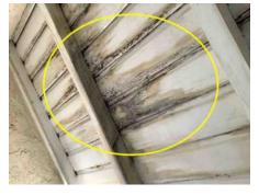
NR 6: Roofing material missing on patio roof
