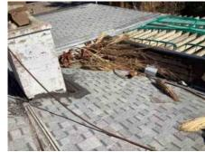
**NB** 16: Nails/Fasteners are protruding from the roof surface. Recommend the entire roof be evaluated and repaired by a qualified Roofing Contractor
