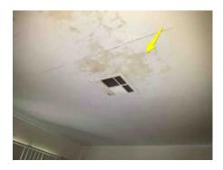
**VR** 47: Stains noted to ceiling in rear room, roof appears to be leaking. We recommend further review and repairs by a qualified specialist in the appropriate trade.
