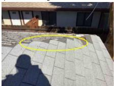
NR 17: Debris should be removed from roof, Recommend further review and repair by a qualified Roofing Contractor
