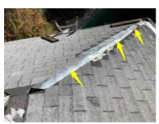
NR 19: Repairs appear to be substandard. Recommend the entire roof be evaluated and repaired by a qualified Roofing Contractor
