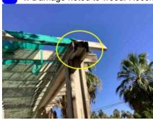
**5:** Moisture damage noted to front porch roof sheathing, Recommend further evaluation by a qualified Termite Company
