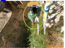
NR 35: Sprinkler main supply line shut off valve handle leaking at front
