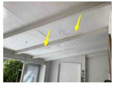
**48:** Ceiling panels separating, damaged and missing in rear room. We recommend further review and repairs by a qualified specialist in the appropriate trade.
