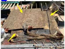
NR 7: Improper installation at patio roof.
