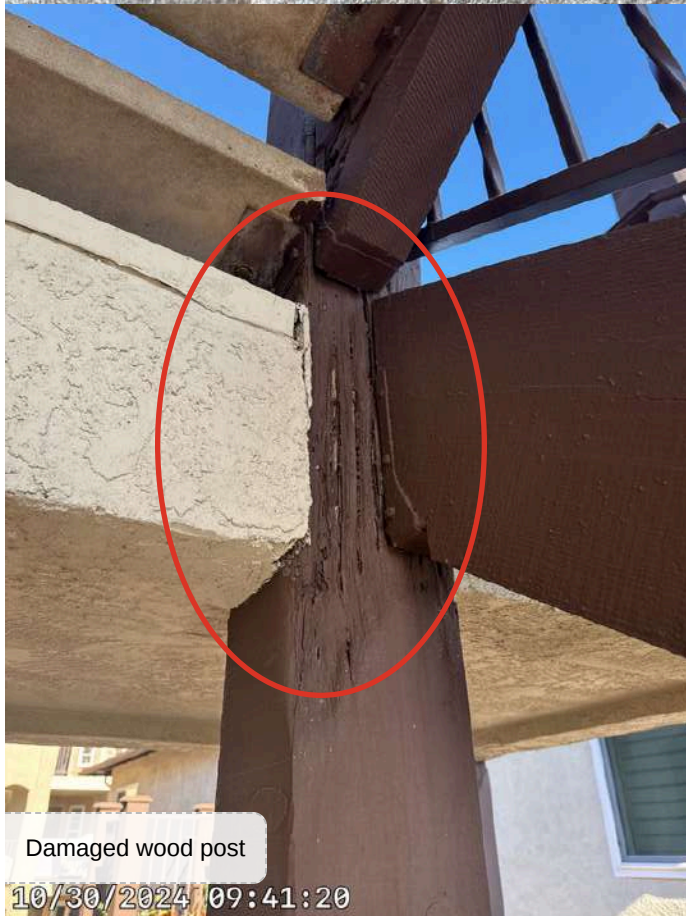
Damaged wood post/support
