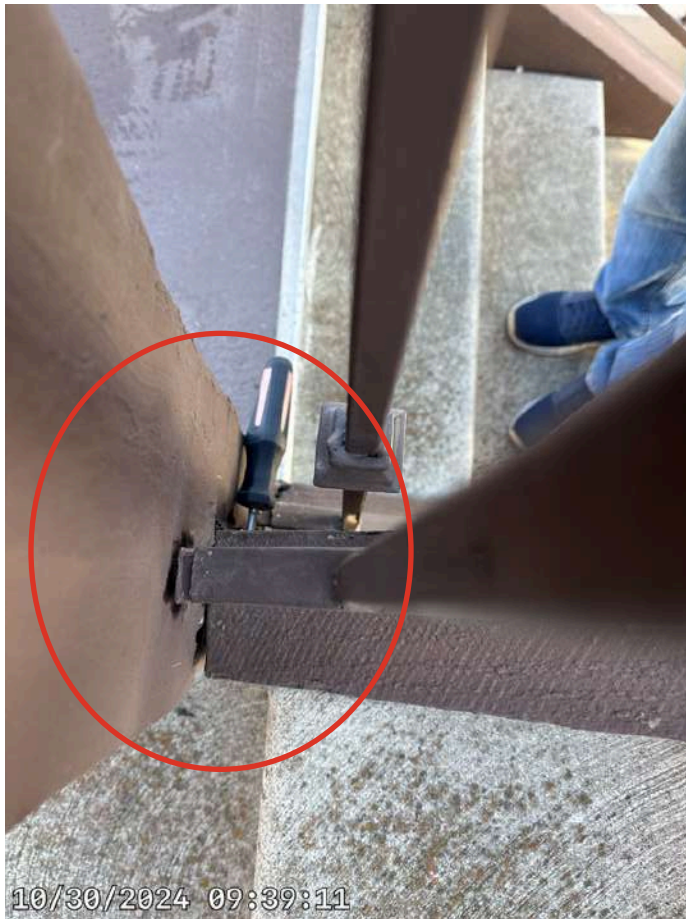
Damage to wood post
