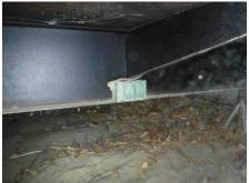
**23:** Loose junction box and conduit with exposed wiring noted. Recommend further review and repair by qualified Electrical Contractor. Repair was completed as requested.
