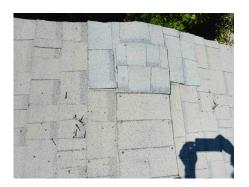
**6:** Nails/Fasteners are protruding from the roof surface. Recommend the entire roof be evaluated and repaired by a qualified Roofing Contractor. Repair was completed as requested.
