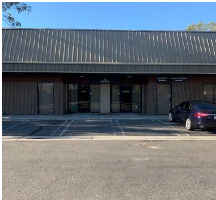
Building Rear Parking
