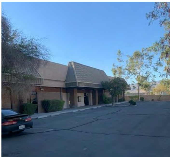
Building Rear Parking
