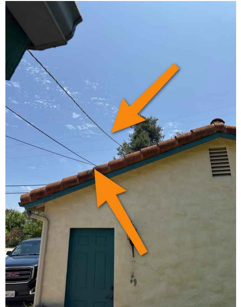
Wires resting on roof of detached garage
