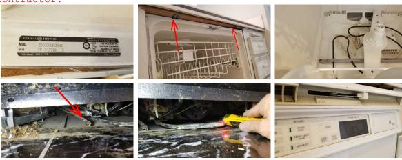
11. Main floor Kitchen Oven: Electric- Oven is missing an anti-tip bracket. This is a safety hazard. Item(s) warrant attention & repair.
