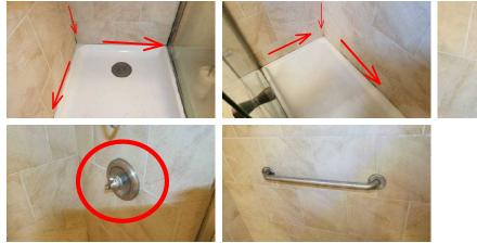
27. Hallway Bathroom Bathroom Enclosure: Hallway Bathroom- Corrosion on the enclosure / door. Caulking needed @ doors / enclosure. Item/s warrant attention & repair.
