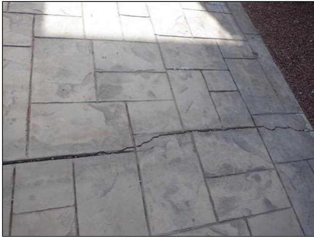
2.4 Item 7(Picture) Walkway Settlement Cracks
