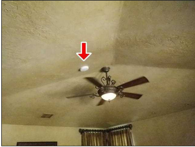
9.7 Item 1(Picture) Smoke Detector To Close To Ceiling Fan
