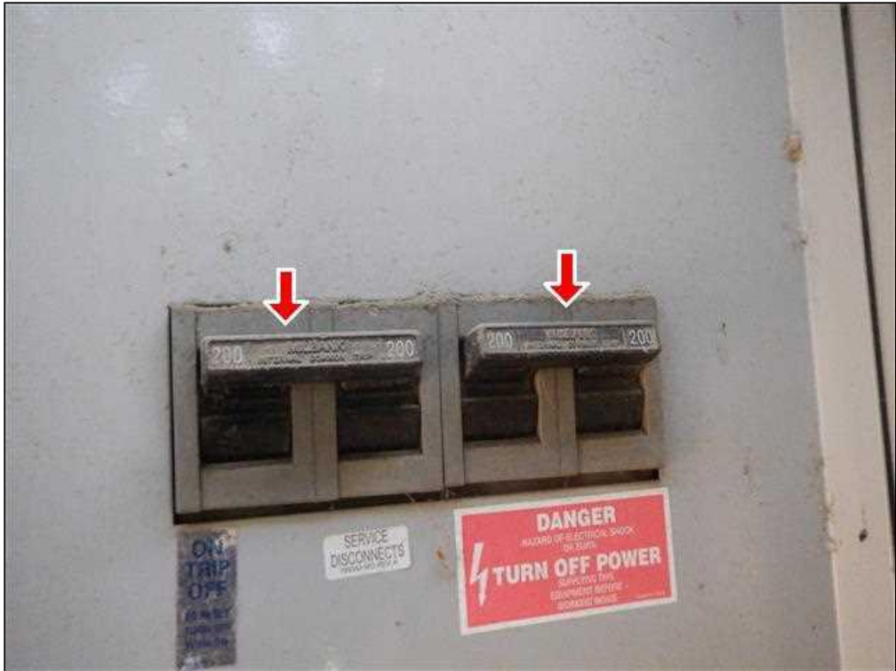
9.1 Item 2(Picture) Main Electrical Panel Disconnects 2 X 200
