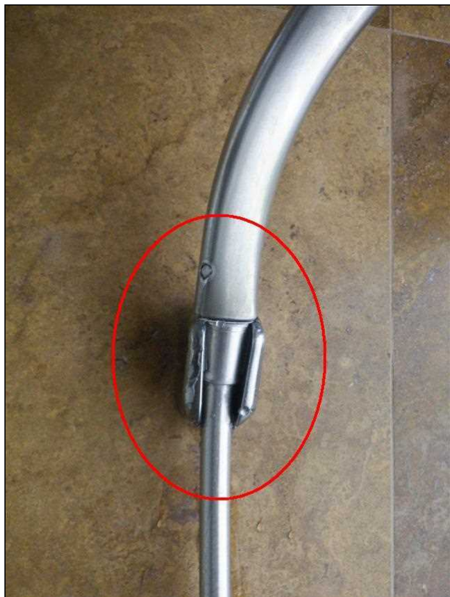
6.4.D Item 1(Picture) Shower Head Fitting Leak
