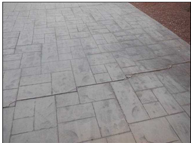
2.4 Item 1(Picture) Driveway Settlement Cracks
