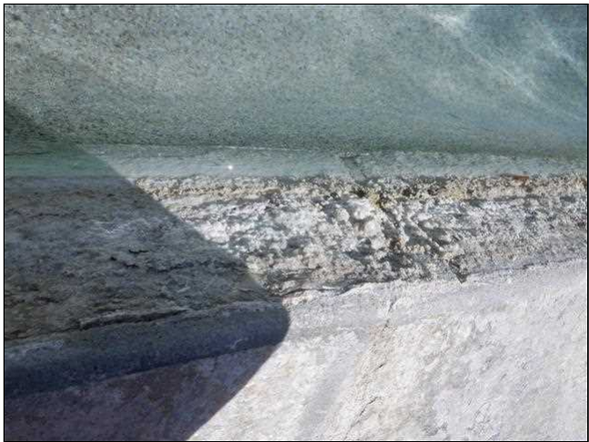
11.13 Item 2(Picture) Pool/Spa Stone Calcium Build Up
