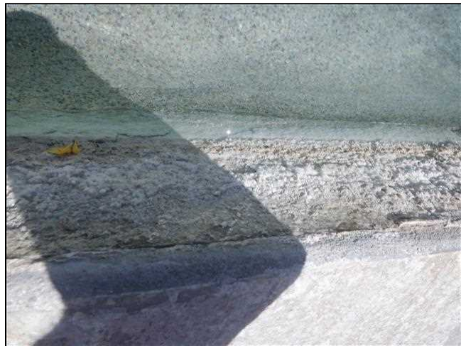
11.13 Item 3(Picture) Pool/Spa Stone Calcium Build Up
