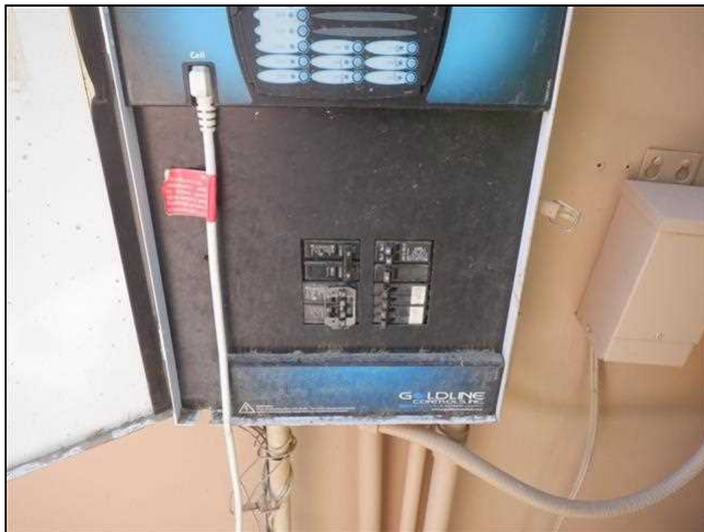
11.26 Item 2(Picture) Controller/Sub Panel Not Bonded
