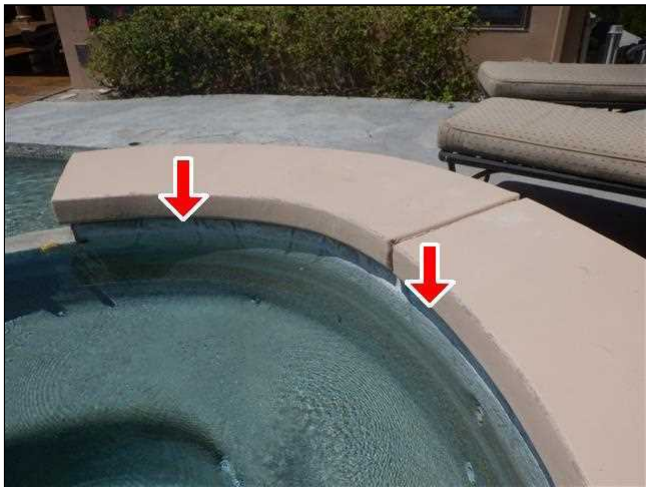
11.13 Item 4(Picture) Pool/Spa Stone Calcium Build Up
