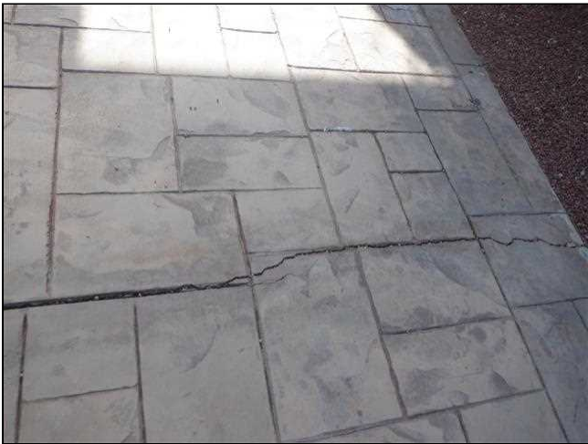
2.4 Item 7(Picture) Walkway Settlement Cracks
