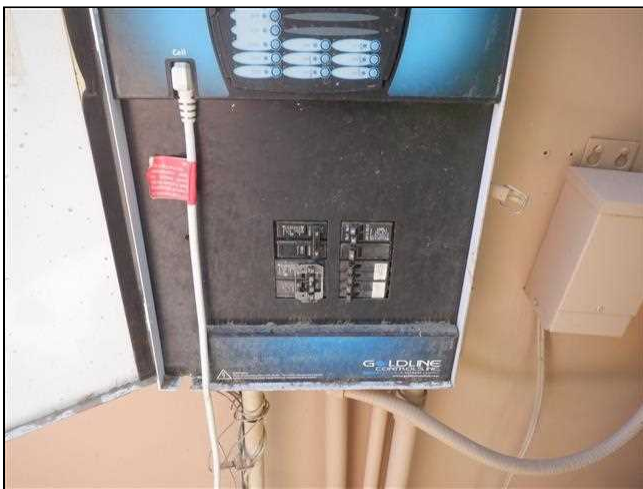
11.26 Item 2(Picture) Controller/Sub Panel Not Bonded
