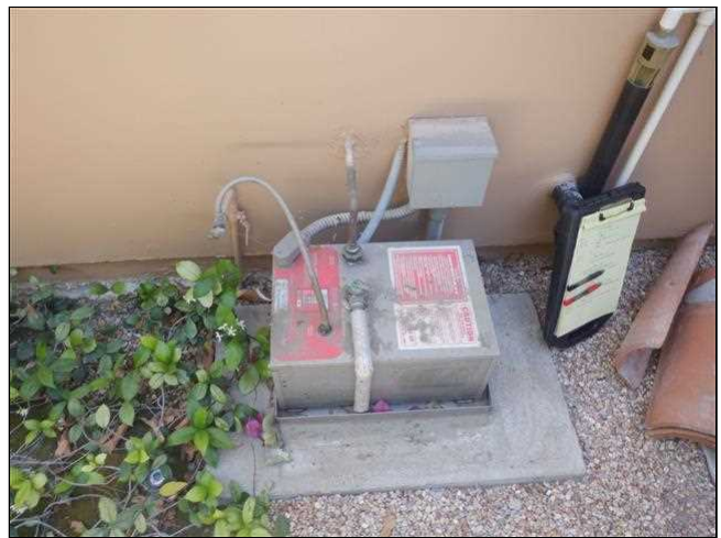
2.17 Item 2(Picture) Misting System Pump 2
