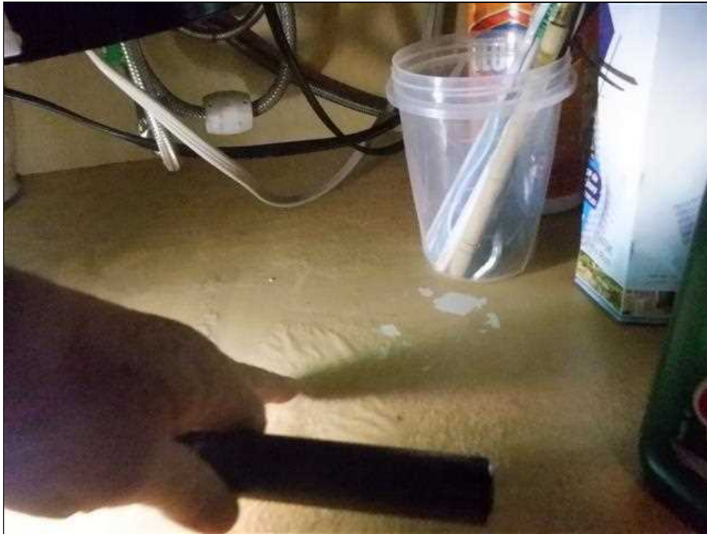
4.5 Item 1(Picture) Main Sink Base Moisture Damage
