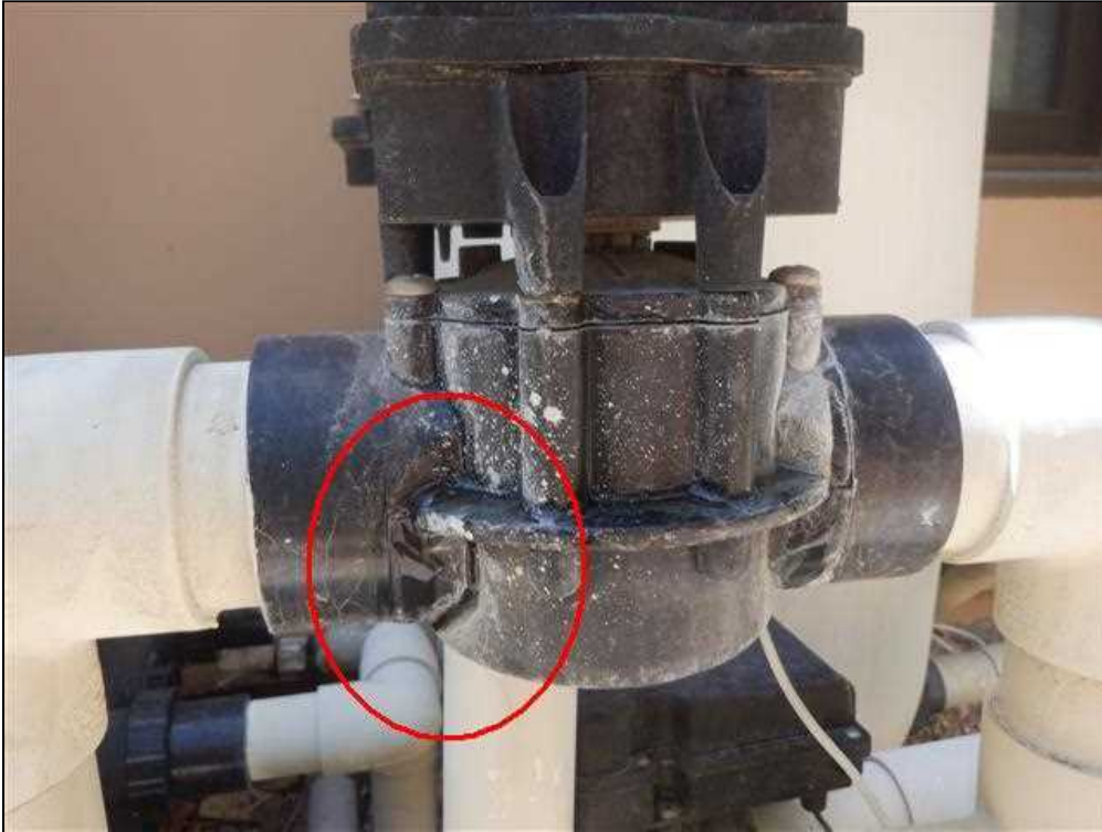
11.9 Item 2(Picture) Actuator Valve Leak
