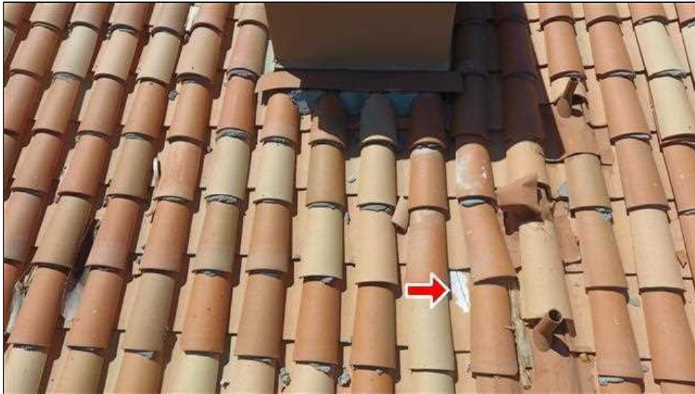
1.0 Item 6(Picture) Damaged Tile
