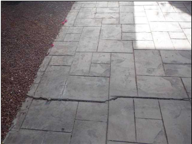
2.4 Item 6(Picture) Walkway Settlement Cracks
