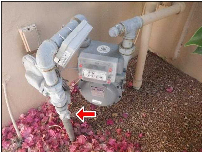
8.6 Item 1(Picture) Main Gas Shut Off
