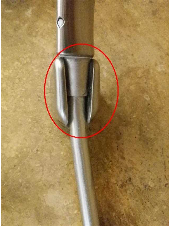
6.3.C Item 1(Picture) Shower Head Fitting Leak
