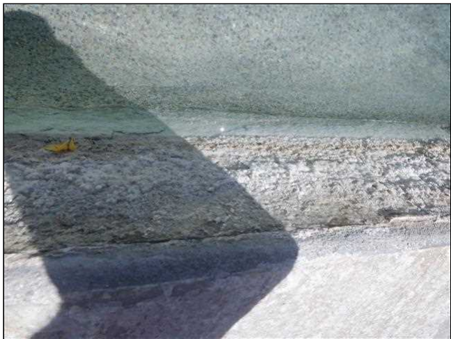
11.13 Item 3(Picture) Pool/Spa Stone Calcium Build Up
