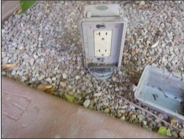
2.7 Item 1(Picture) Upper Courtyard GFCI Failed To Reset
