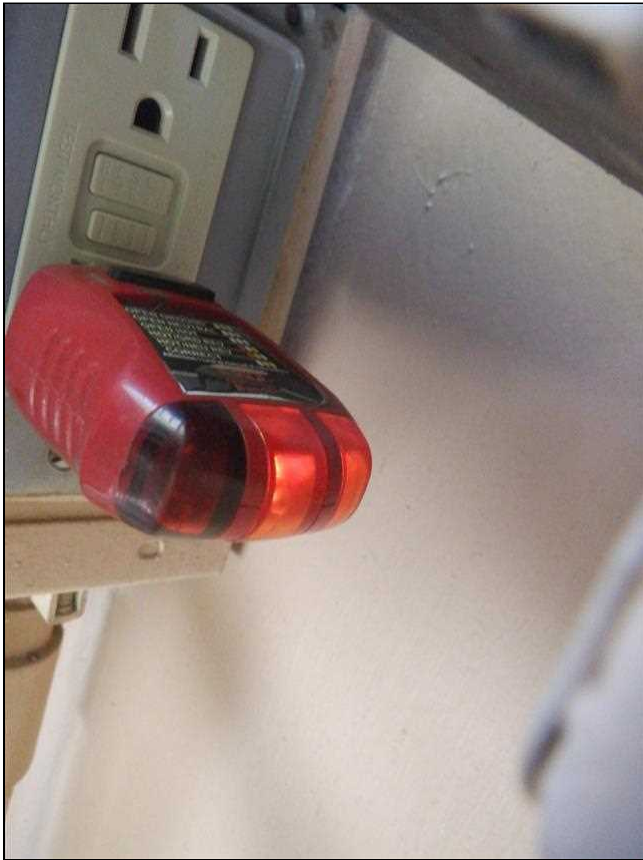
11.16 Item 1(Picture) Pool/Spa Light GFCI Failed To Reset
