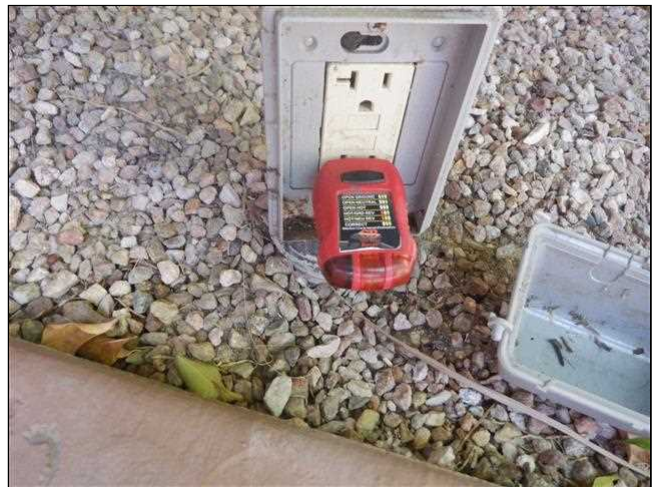
2.7 Item 2(Picture) Upper Courtyard GFCI Failed To Reset
