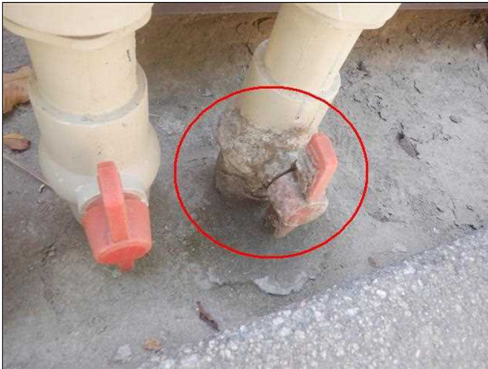
11.9 Item 3(Picture) Plumbing Valve Seepage Noted
