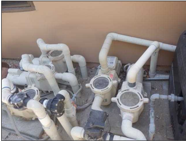
11.17 Item 1(Picture) Pool Pumps/Motors
