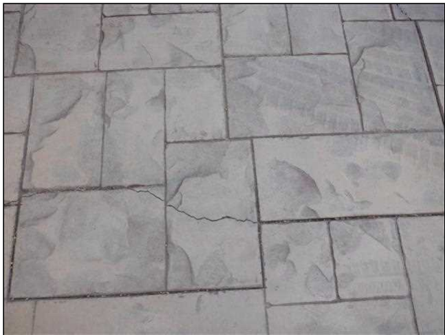
2.4 Item 3(Picture) Driveway Settlement Cracks
