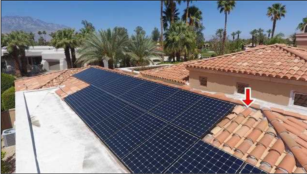
1.0 Item 4(Picture) Damaged Tile
