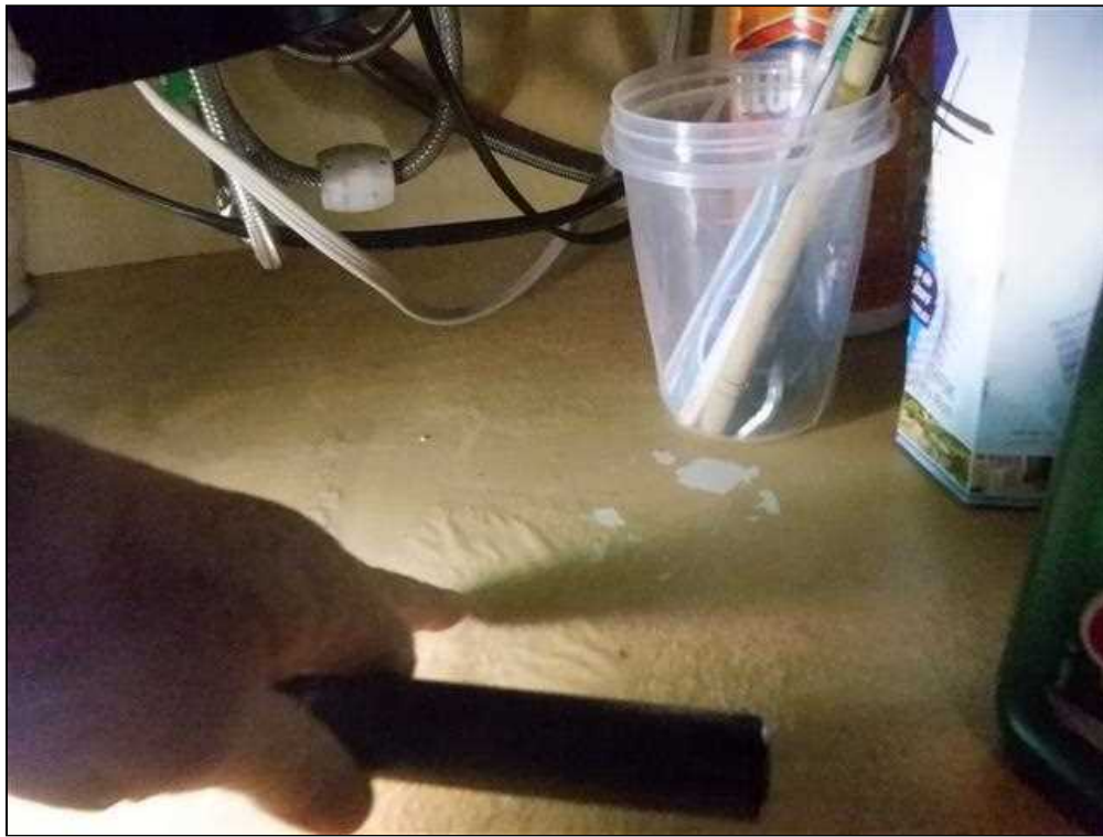
4.5 Item 1(Picture) Main Sink Base Moisture Damage
