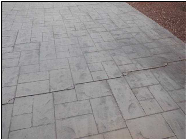
2.4 Item 1(Picture) Driveway Settlement Cracks
