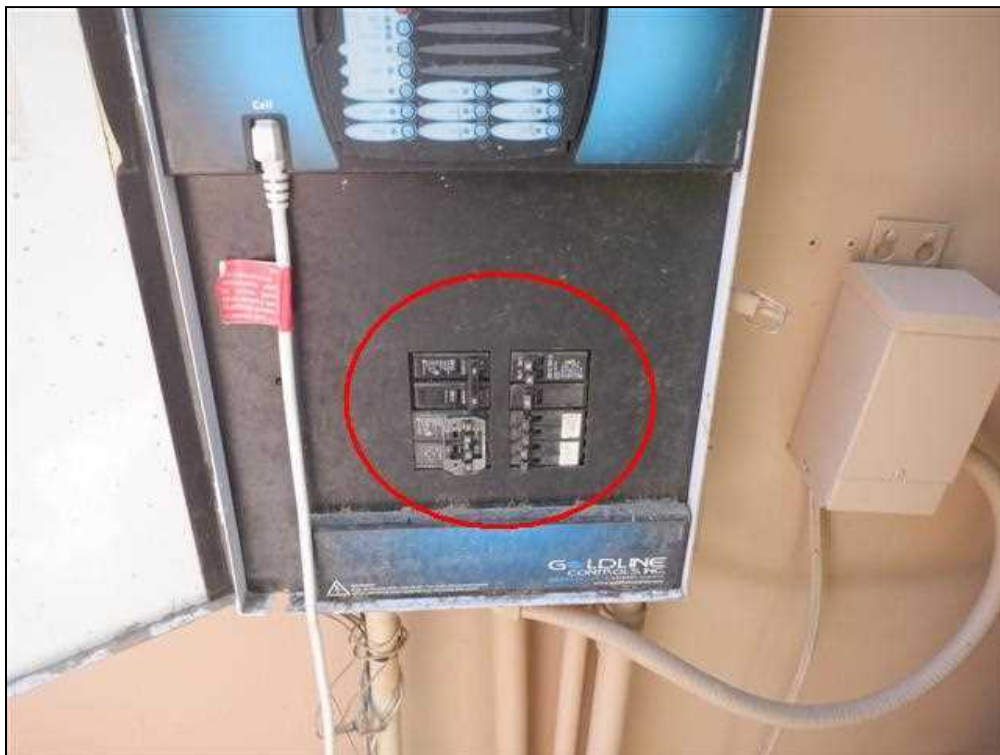
11.26 Item 4(Picture) Pool/Spa Equipment Not GFCI Protected
