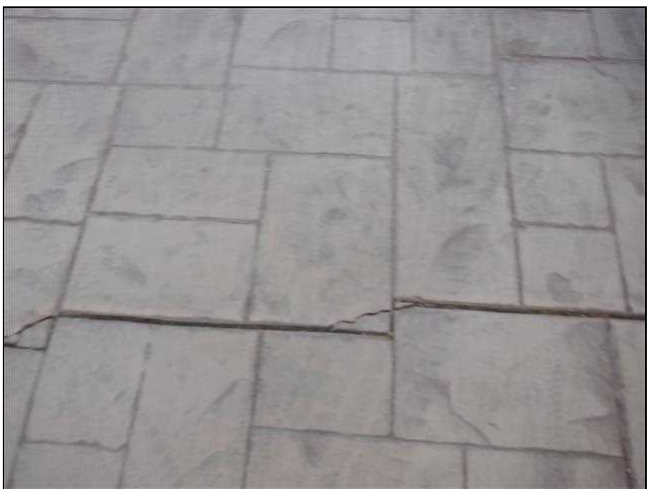
2.4 Item 2(Picture) Driveway Settlement Cracks
