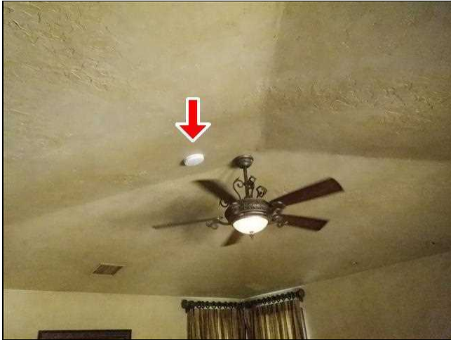
9.7 Item 1(Picture) Smoke Detector Too Close To Ceiling Fan
