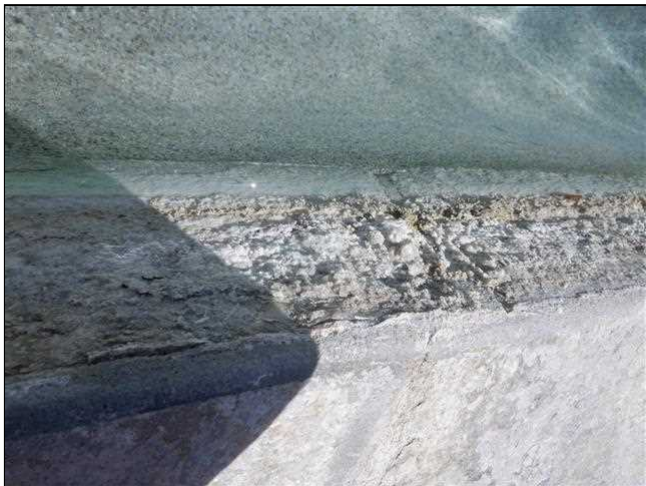
11.13 Item 2(Picture) Pool/Spa Stone Calcium Build Up
