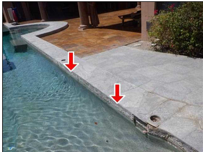
11.13 Item 1(Picture) Pool Stone Calcium Build Up
