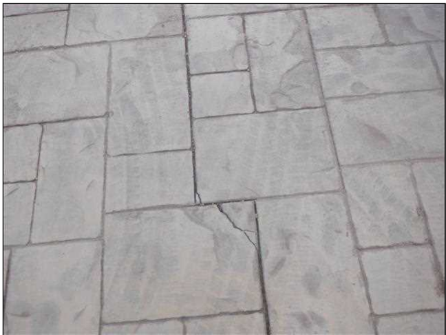
2.4 Item 4(Picture) Driveway Settlement Cracks
