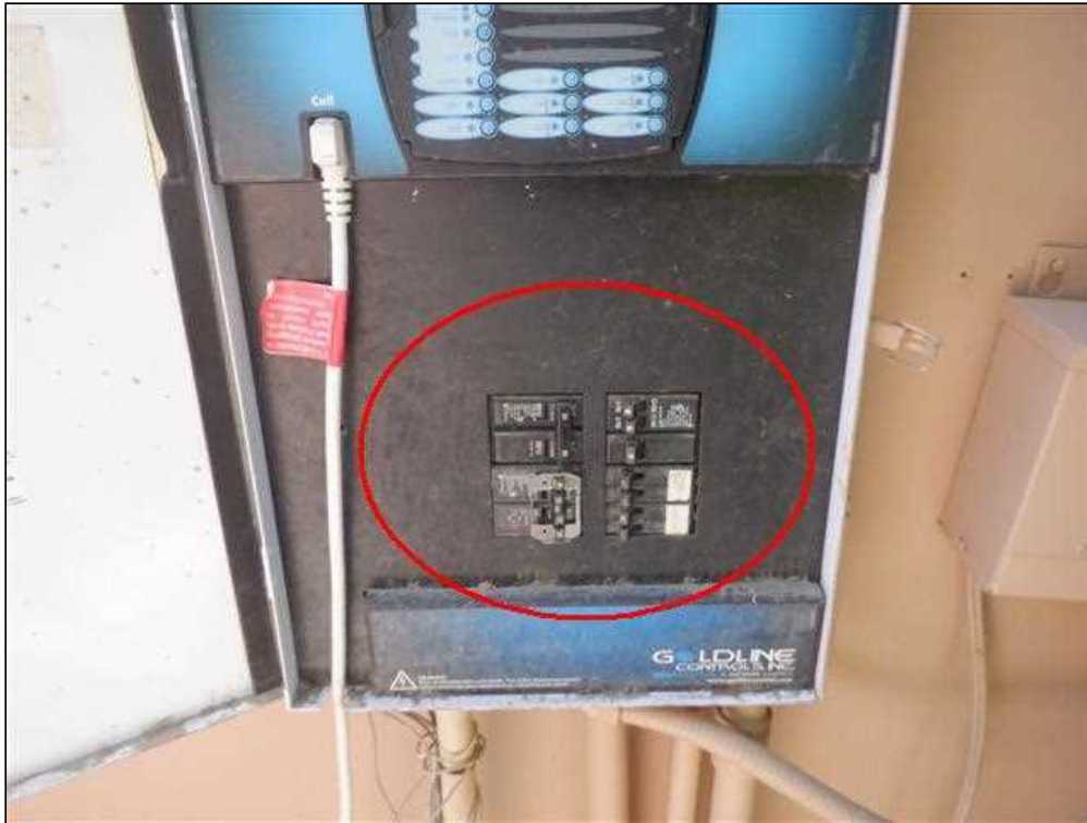
9.1 Item 5(Picture) Pool/Spa Sub Panel Circuits Not Labeled
