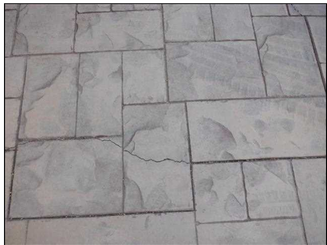
2.4 Item 3(Picture) Driveway Settlement Cracks
