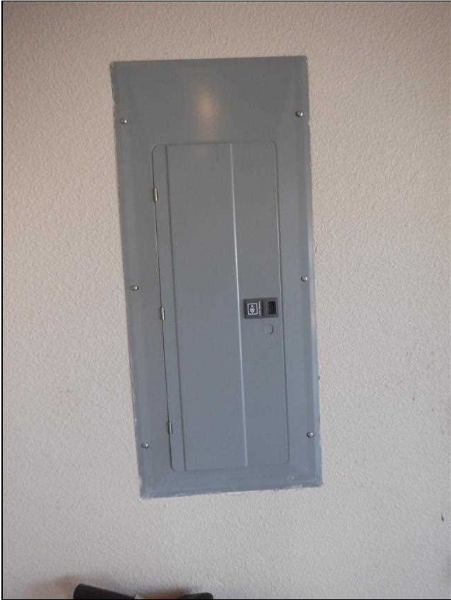
3.10 Item 1(Picture) Electrical Sub Panel
