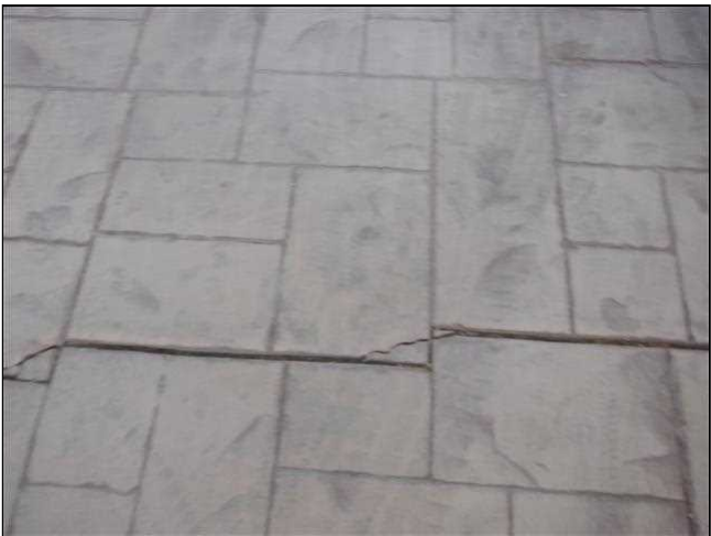
2.4 Item 2(Picture) Driveway Settlement Cracks
