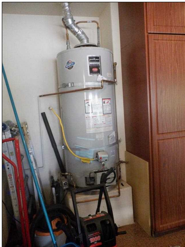
8.3 Item 1(Picture) Water Heater 2 Seismic Straps Only
