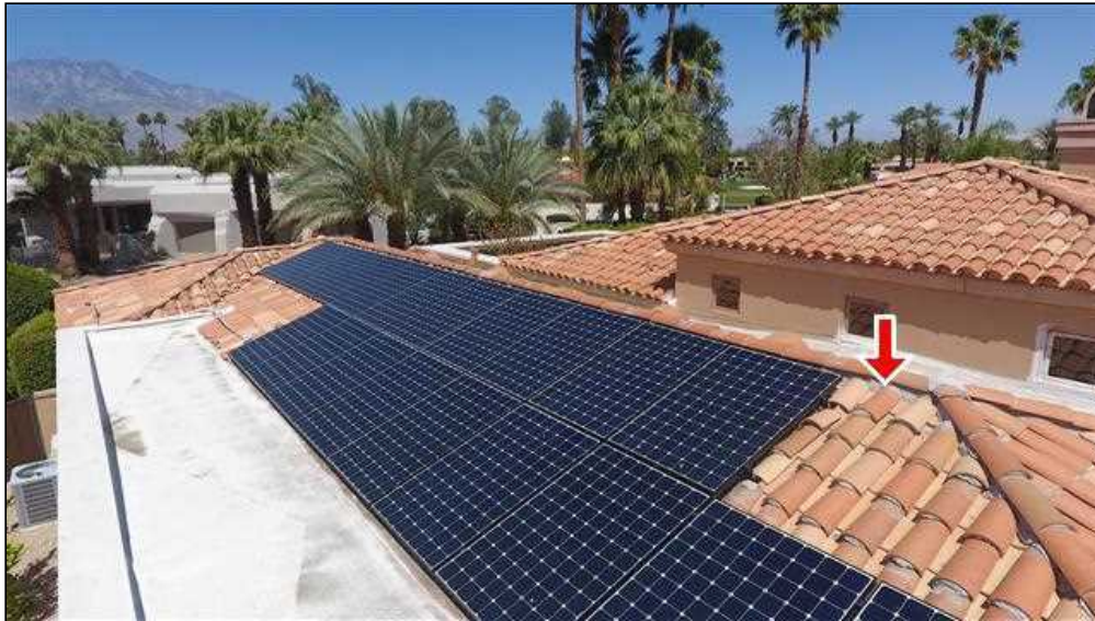
1.0 Item 4(Picture) Damaged Tile
