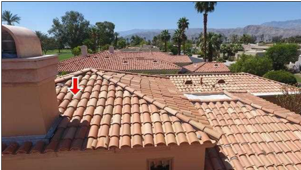
1.0 Item 5(Picture) Damaged Tile
