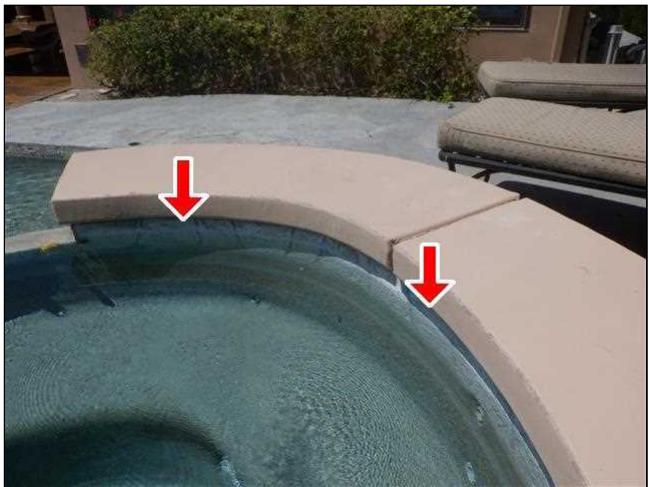
11.13 Item 4(Picture) Pool/Spa Stone Calcium Build Up
