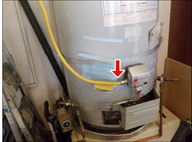
8.2 Item 2(Picture) Water Heater Fuel Line Missing Sediment Trap
