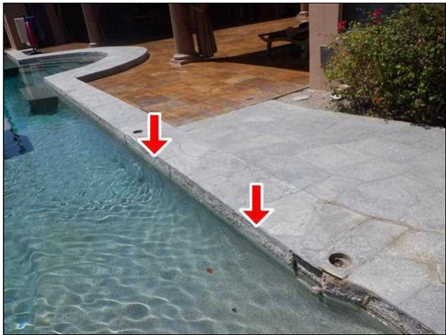
11.13 Item 1(Picture) Pool Stone Calcium Build Up
