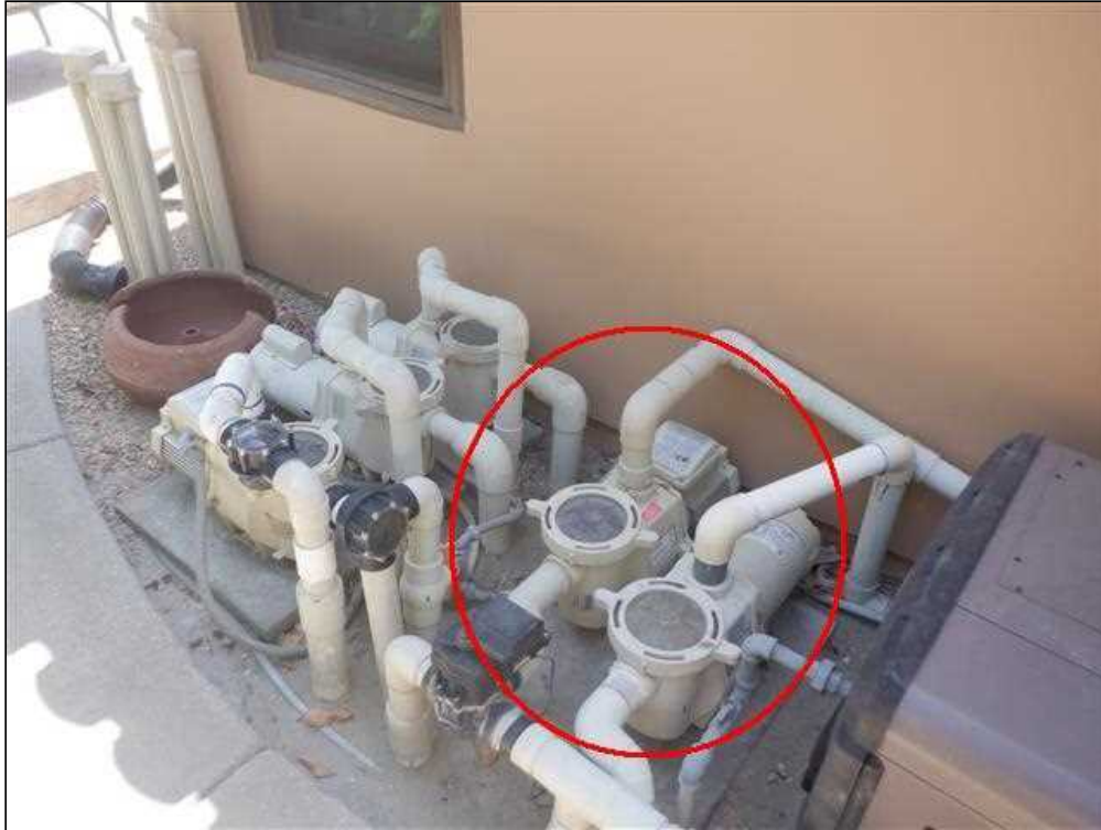
11.26 Item 1(Picture) Pumps Not Bonded
