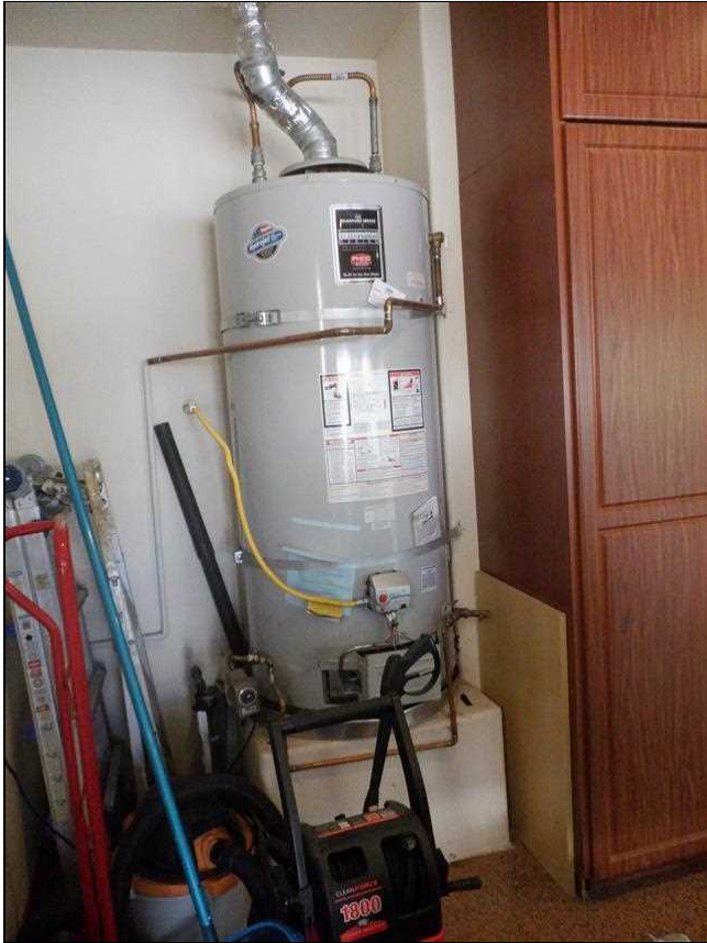
8.3 Item 1(Picture) Water Heater 2 Seismic Straps Only
