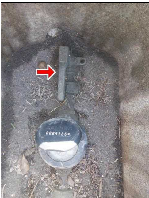
8.4 Item 3(Picture) Main Water Shut Off
