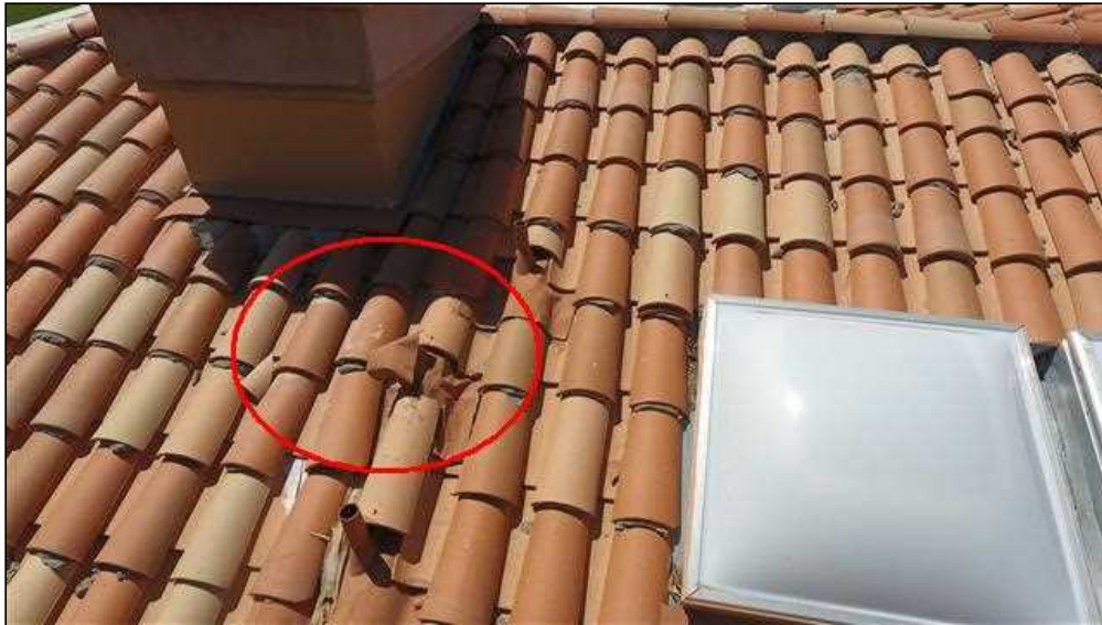
1.0 Item 2(Picture) Damaged Tile
