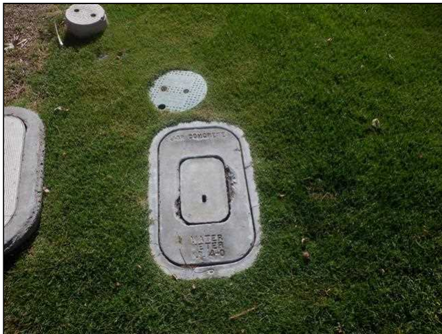
8.4 Item 2(Picture) Main Water Shut Off
