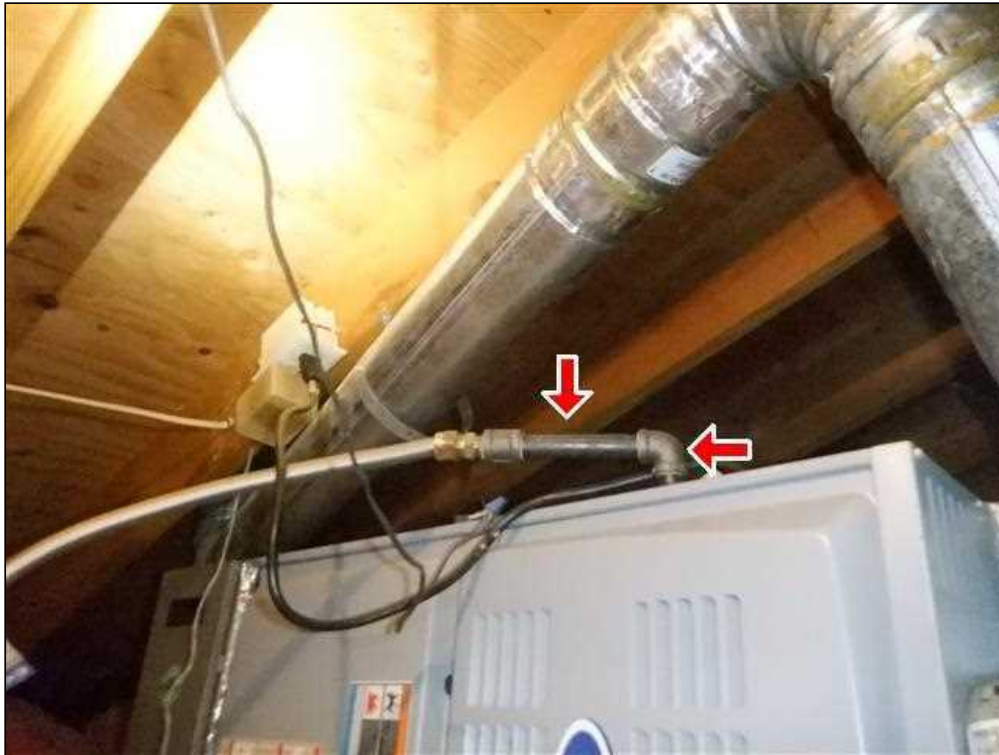
10.0.A Item 2(Picture) Heating Unit South Fuel Line Missing Sediment Trap
