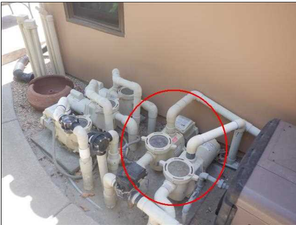
11.26 Item 1(Picture) Pumps Not Bonded
