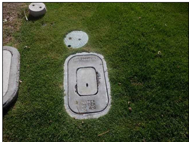
8.4 Item 2(Picture) Main Water Shut Off
