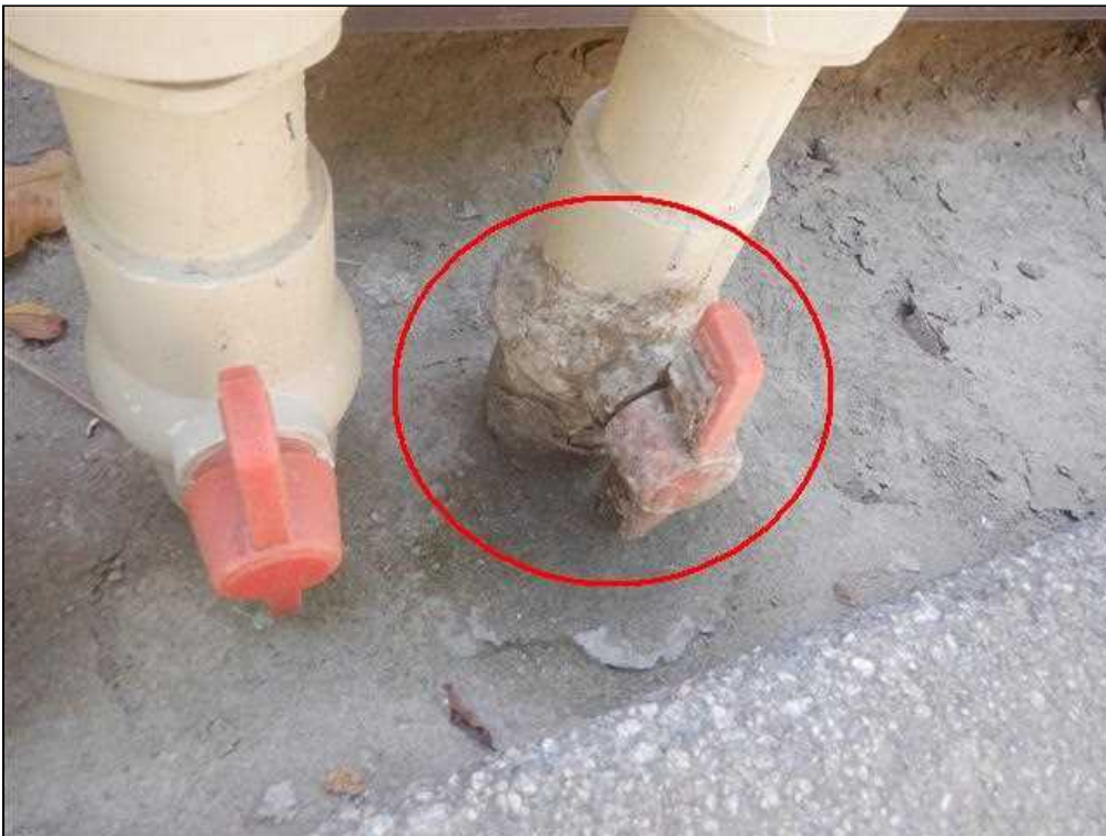
11.9 Item 3(Picture) Plumbing Valve Seepage Noted
