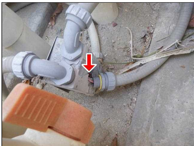
11.26 Item 3(Picture) Loose Conduit/Exposed Wires
