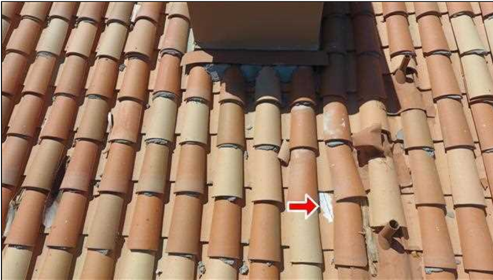
1.0 Item 6(Picture) Damaged Tile
