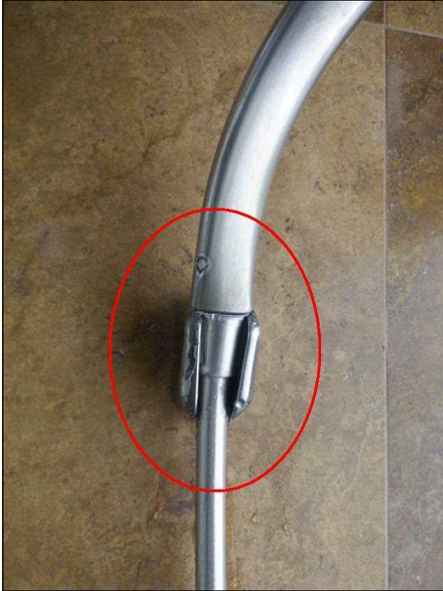
6.4.D Item 1(Picture) Shower Head Fitting Leak
