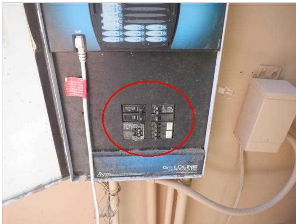
11.26 Item 4(Picture) Pool/Spa Equipment Not GFCI Protected
