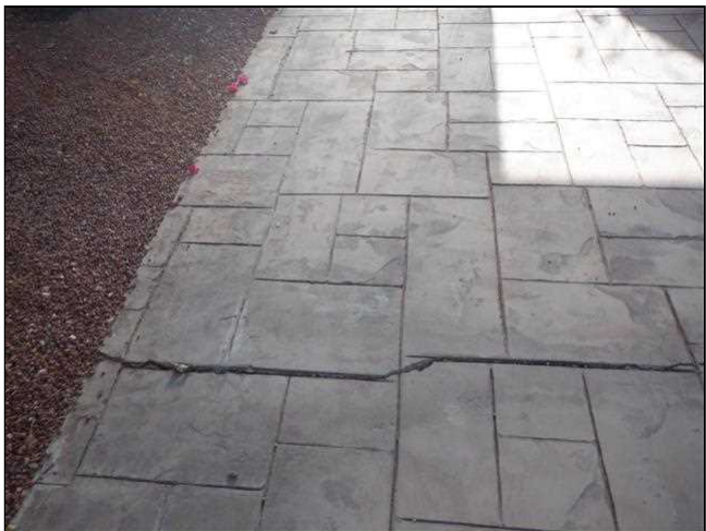
2.4 Item 6(Picture) Walkway Settlement Cracks
