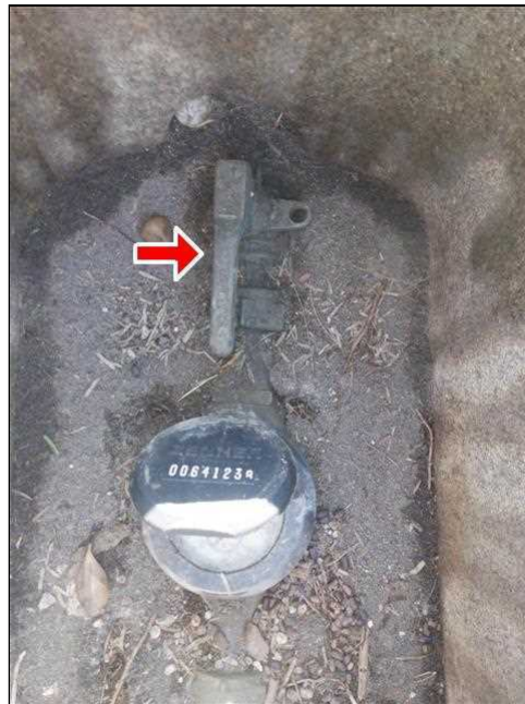
8.4 Item 3(Picture) Main Water Shut Off
