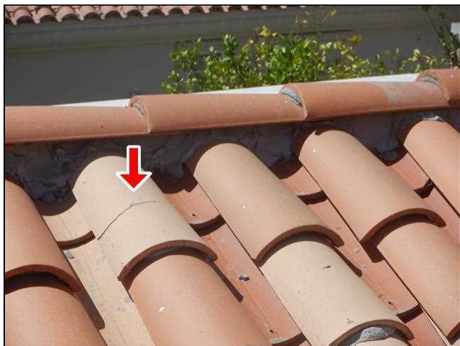
1.0 Item 1(Picture) Damaged Tile
