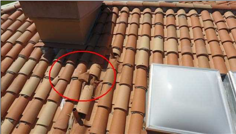
1.0 Item 2(Picture) Damaged Tile
