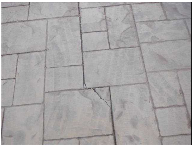
2.4 Item 4(Picture) Driveway Settlement Cracks
