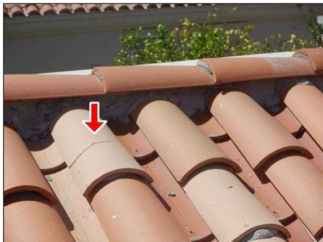
1.0 Item 1(Picture) Damaged Tile
