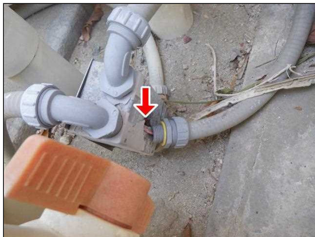
11.26 Item 3(Picture) Loose Conduit/Exposed Wires
