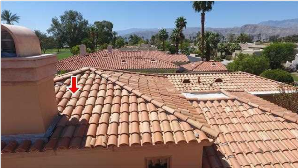
1.0 Item 5(Picture) Damaged Tile
