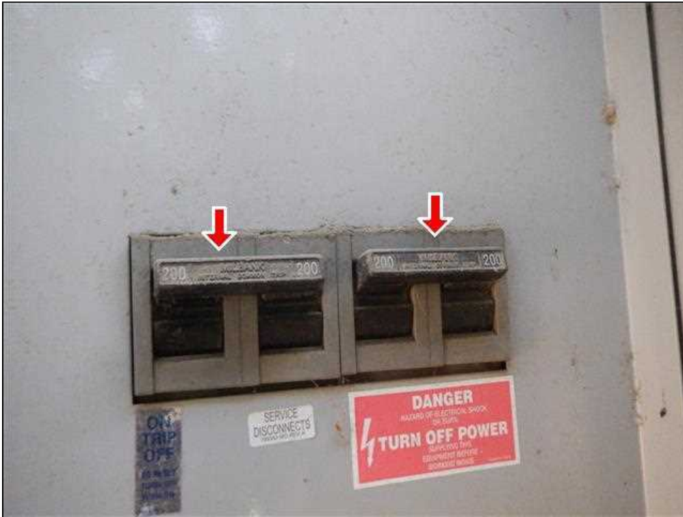
9.1 Item 2(Picture) Main Electrical Panel Disconnects 2 X 200
