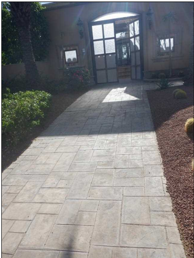
2.4 Item 5(Picture) Walkway Settlement Cracks
