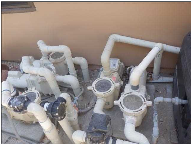
11.17 Item 1(Picture) Pool Pumps/Motors
