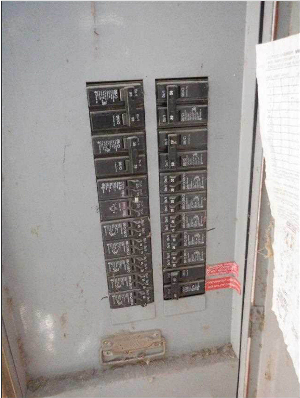
9.1 Item 3(Picture) Main Electrical Panel Distribution Missing Labels
