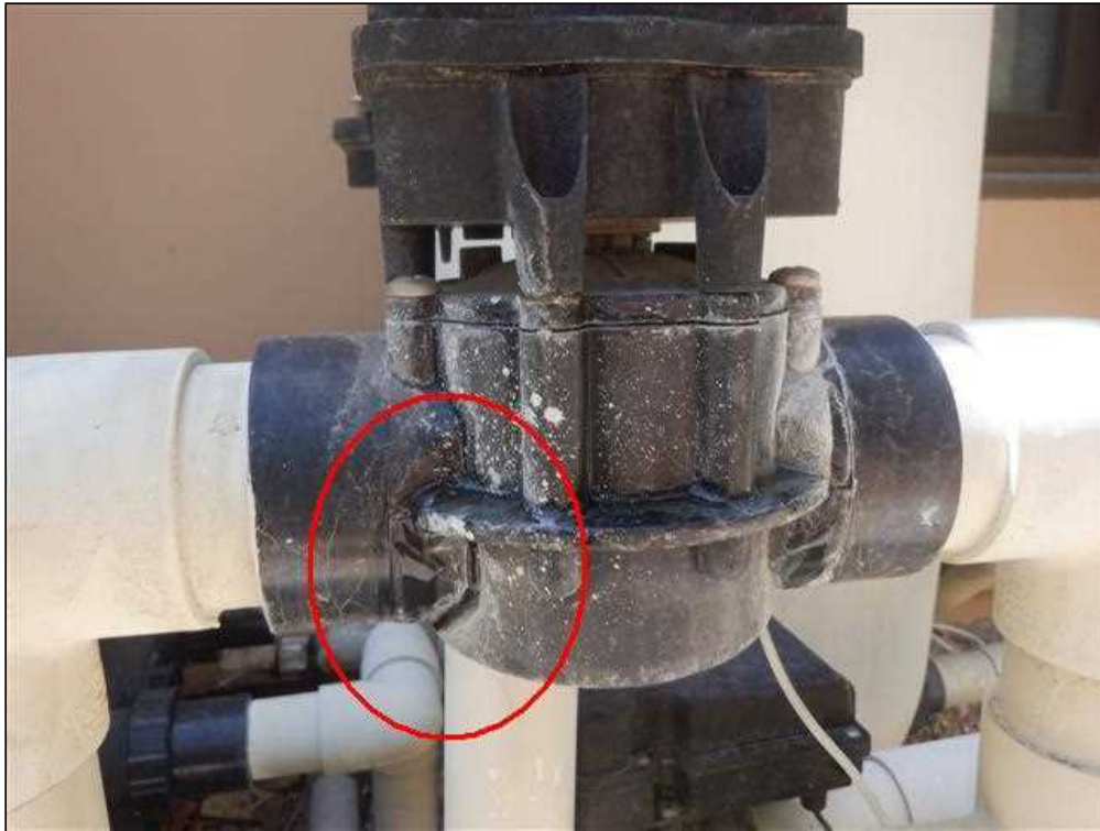
11.9 Item 2(Picture) Actuator Valve Leak
