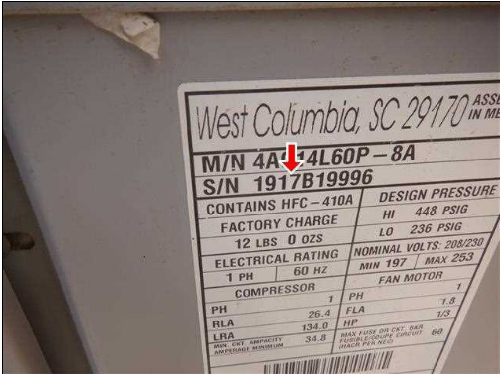
10.5.A Item 2(Picture) Cooling Unit South MFG Date 2017
