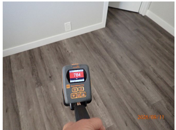
Elevated moisture readings on floor in guest bedroom
