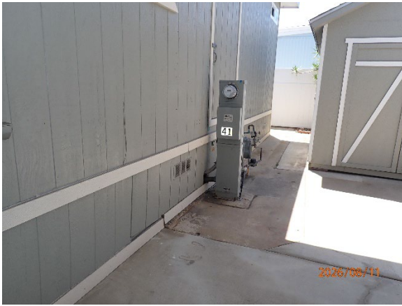
Perimeter vents at north side of home below primary ensuite bathroom
