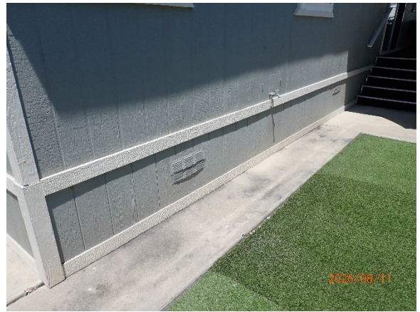
Perimeter vents at south side of home below primary bedroom
