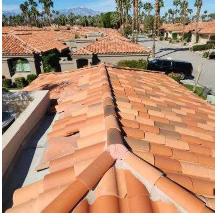
Garage Roof GV
