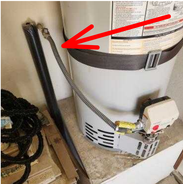
Missing sediment trap on gas supply pipe to water heater-NTBS
