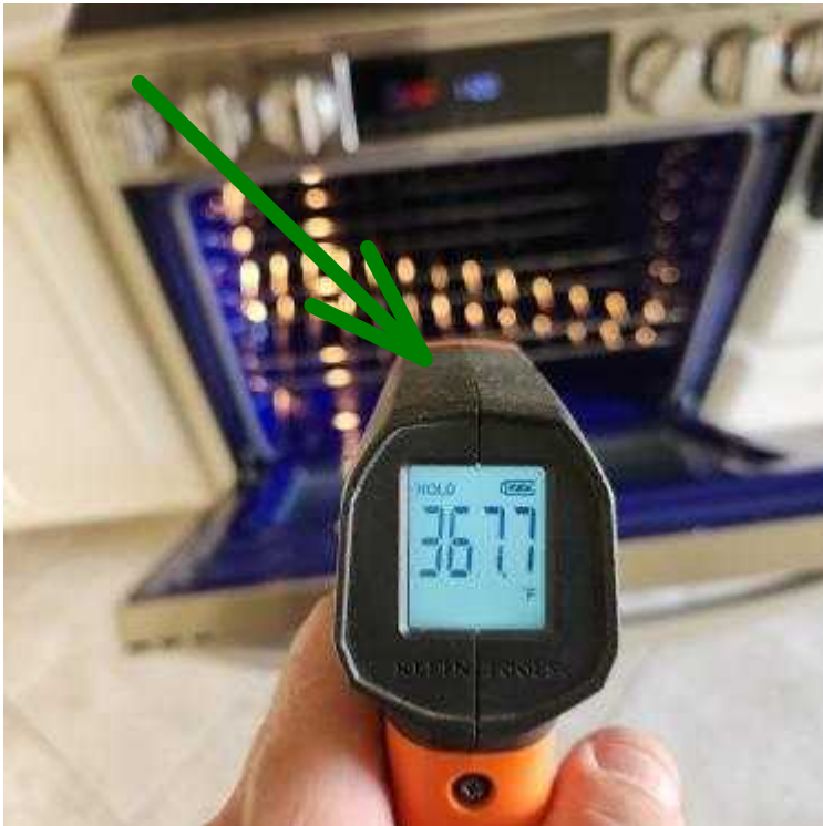
Electric oven in kitchen operated at time of inspection (LG)
