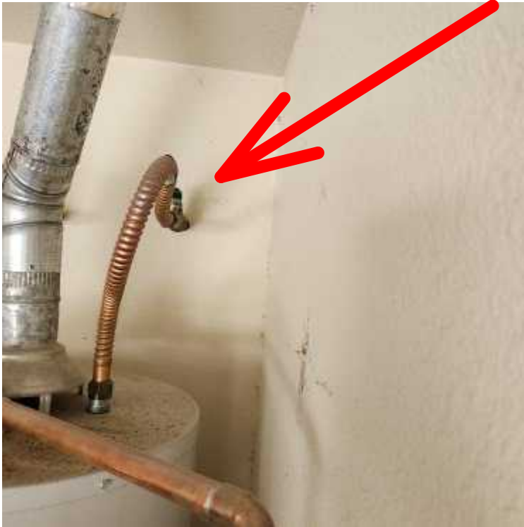
Missing thermal expansion tank on plumbing to water heater-NTBS
