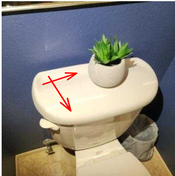
Cracked lid on north bathroom toilet tank
