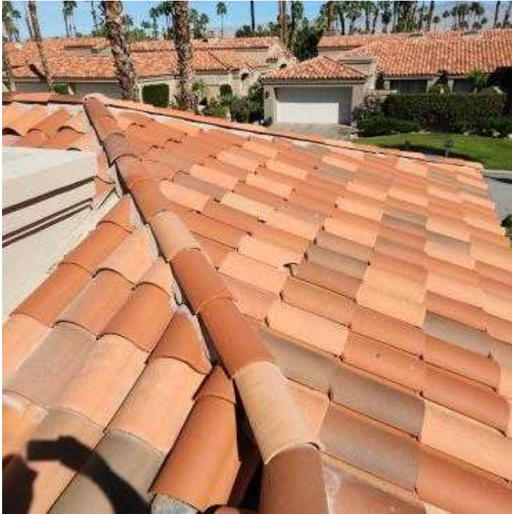
Garage Roof GV
