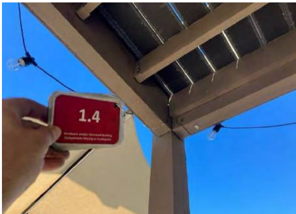
1143 Via Cuesta, Balcony, West 1.4 Hardware and/or Structural Building Component Issues
