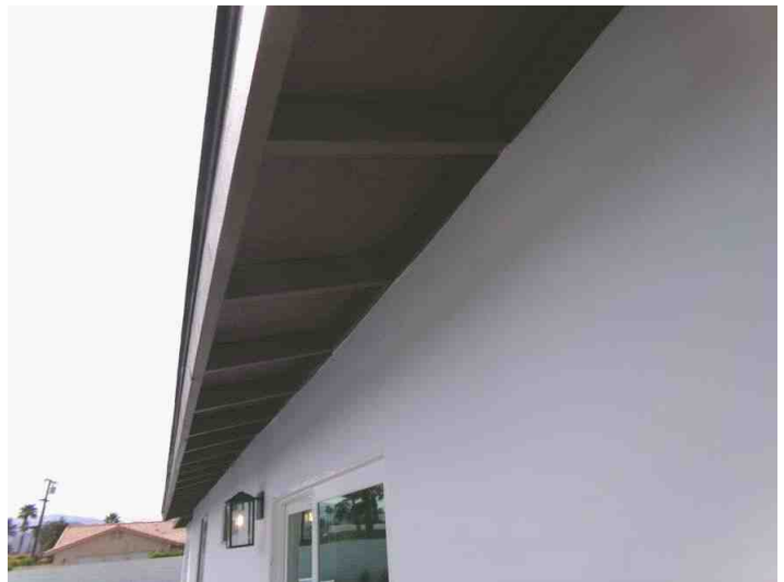
NEW EXTERIOR PAINT
