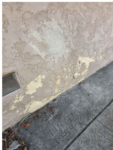
Left of building
