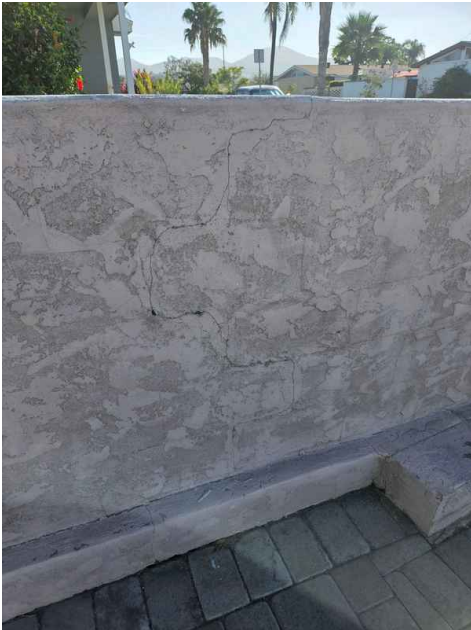
Front of building
