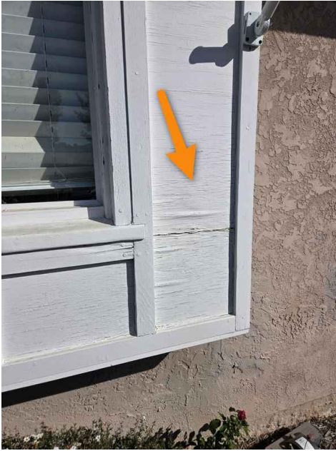
Front of building
