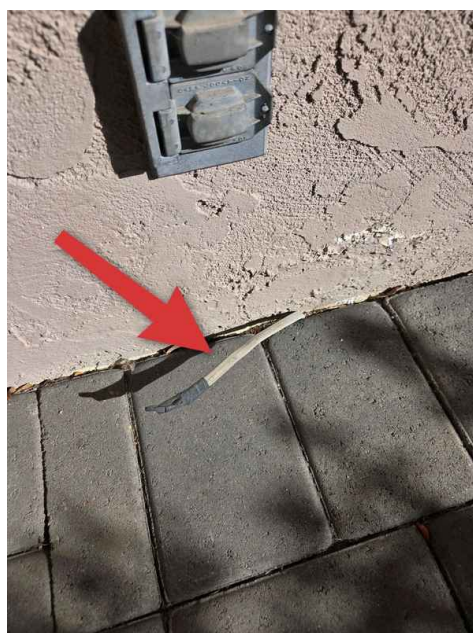
Front of building
