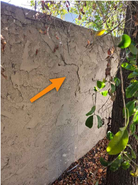
Right of building
