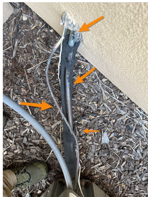
HVAC Refrigerant Pipes
