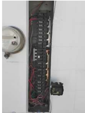
Missing Circuit Labels
