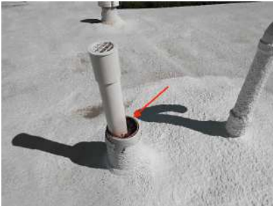
Inadequate Seal/Waterproofing
