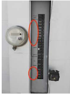
Missing Circuit Labels
