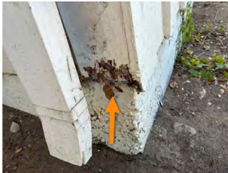
Rear of Property Garage
