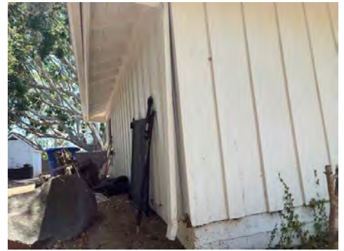
Rear of Property Garage
