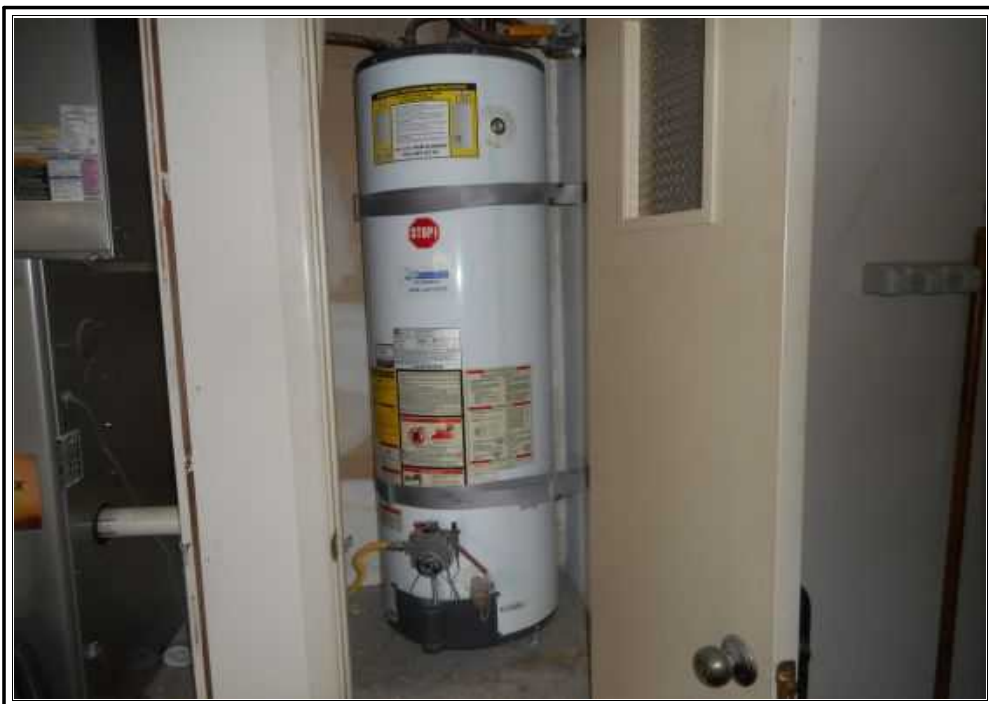
Hot Water Heater is double strapped.
