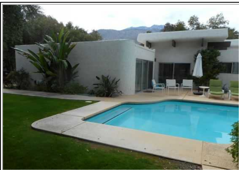
REAR EAST-SOUTH SIDE
