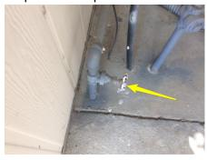
28: There is an uncapped gas valve in the the laundry area. If it remains unused, we recommend it be capped to reduce the chance of gas leakage.
