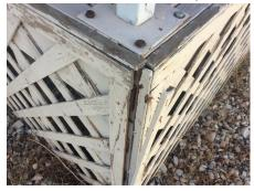
**s-16:** If caulking is needed for maintenance, or in preparation for the next paint job, we suggest a high quality urethane sealant such as 'Sikaflex'. Latex, butyl, oil based, silicone or 'architectural grade' sealants should be avoided on the exterior.
