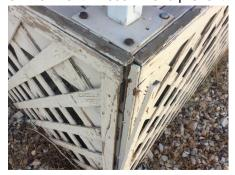
**16:** If caulking is needed for maintenance, or in preparation for the next paint job, we suggest a high quality urethane sealant such as 'Sikaflex'. Latex, butyl, oil based, silicone or 'architectural grade' sealants should be avoided on the exterior.
