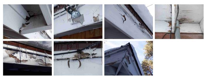
Wood damage noted at various locations of the eaves. Confirm with termite control co before the close of escrow.
