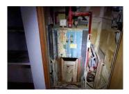
Lack of a proper platform in front of the unit. One should have at least a 30" inch platform to meet proper requirements. Recommend improvement.
