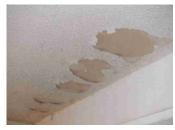
Acoustic type ceiling noted. Ceiling may contain asbestos type material. Recommend consulting with an abatement contractor for further evaluation if desired.
