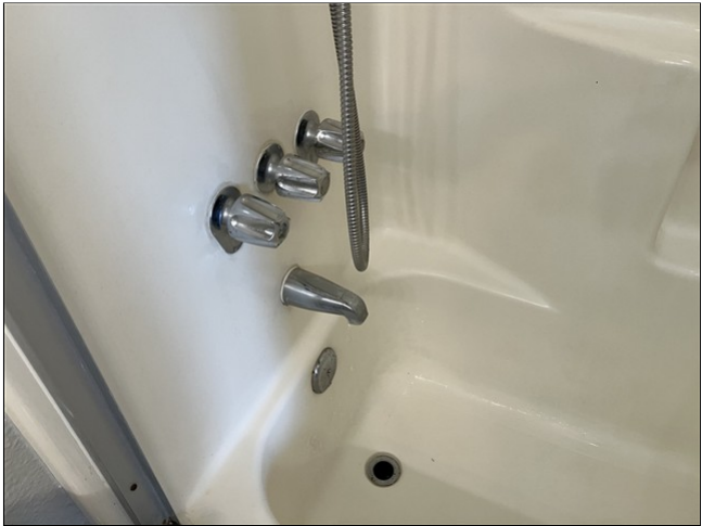
6.5 Item 5(Picture) shower: aged shower valves observed
