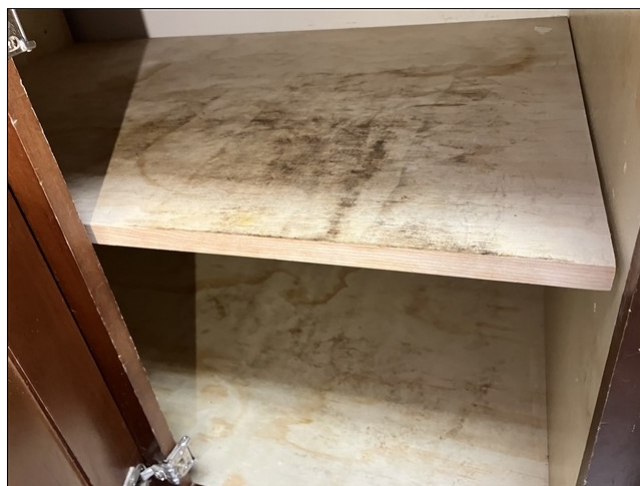
4.4 Item 8(Picture) kitchen cabinet: stains visible at cabinet shelf and base
