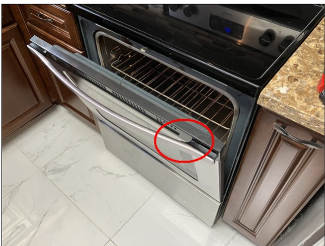
10.1 Item 2(Picture) loose handle / missing anti-tip bracket
