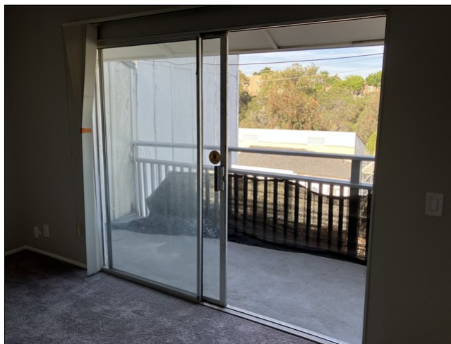
2.1 Item 2(Picture) bedroom slider appeared aged as was difficult to operate
