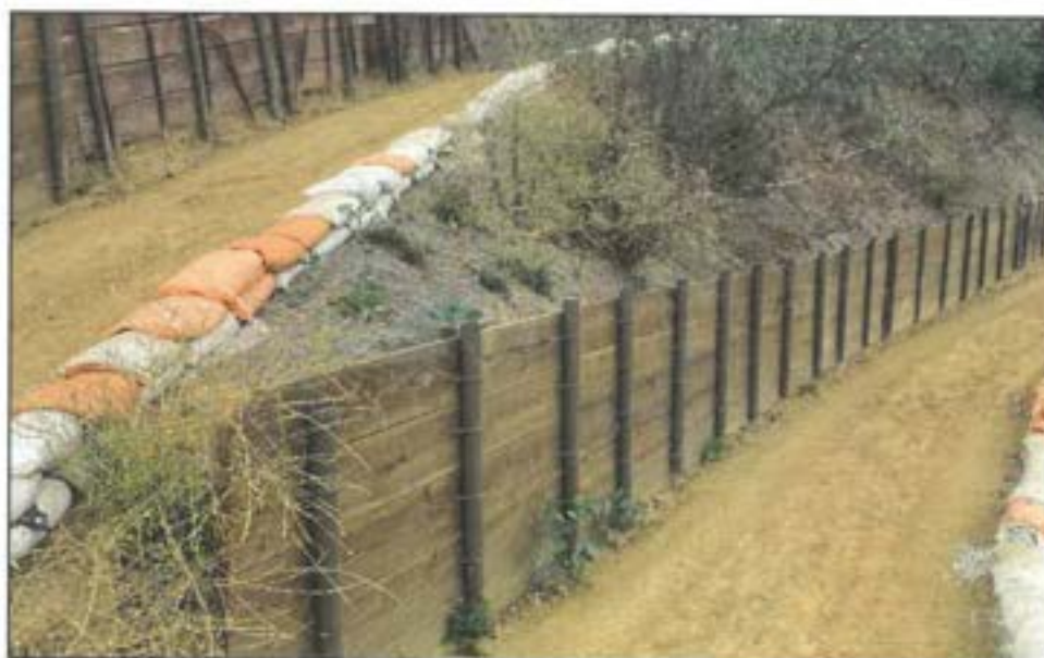
Access Road with Erosion Control
