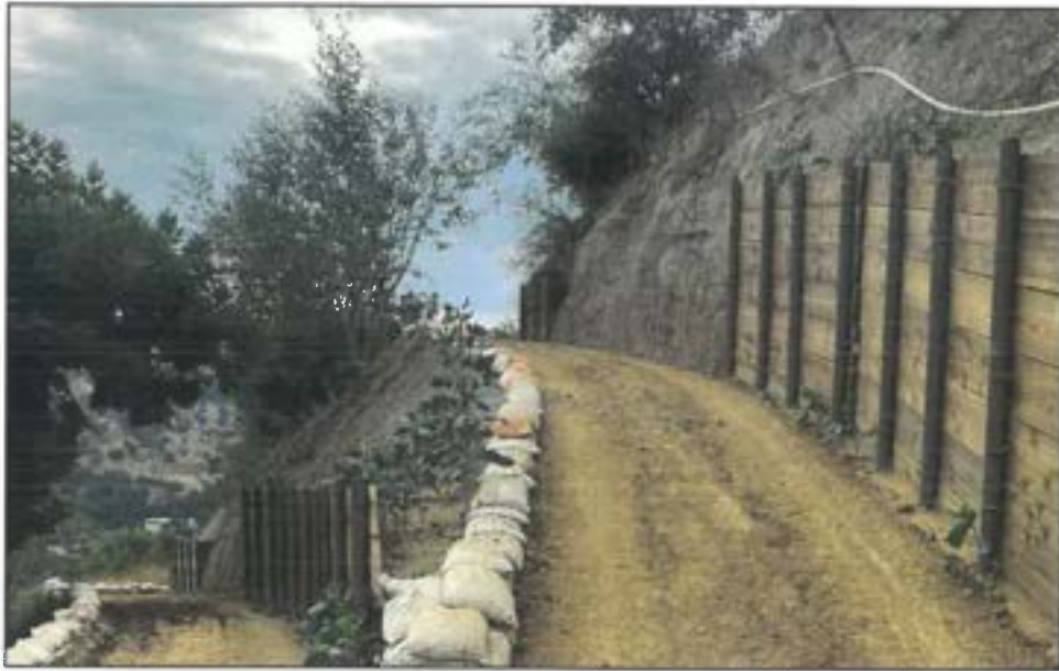
Access Road with Erosion Control
