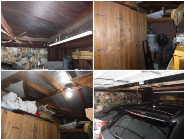
Stored items restricted viewing of the garage interior.
