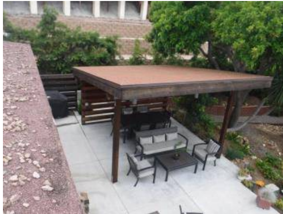
Detached, Wood framing.
