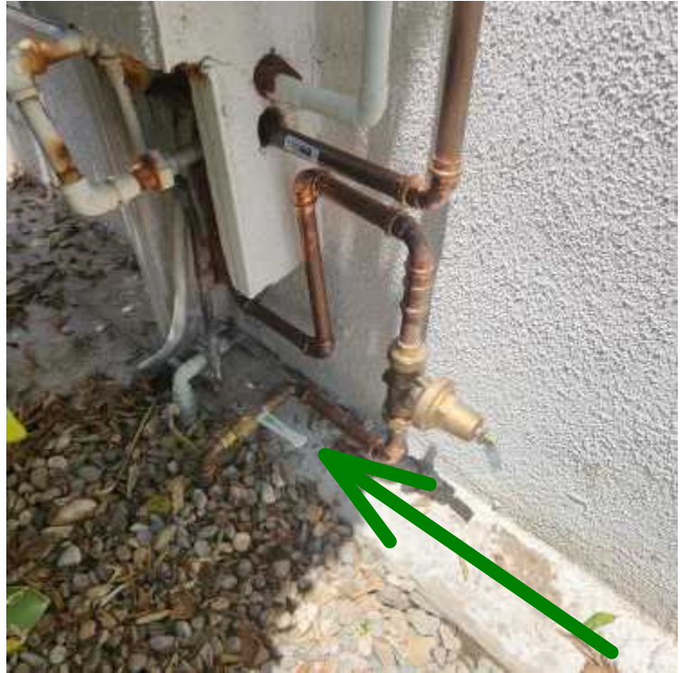
Water shut off to house operated (Located on south side of house)
