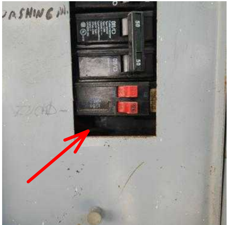
Interior cover to electrical panel missing knockout insert
