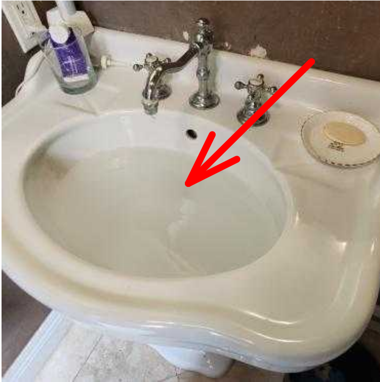
Sink in north bathroom drains slow
