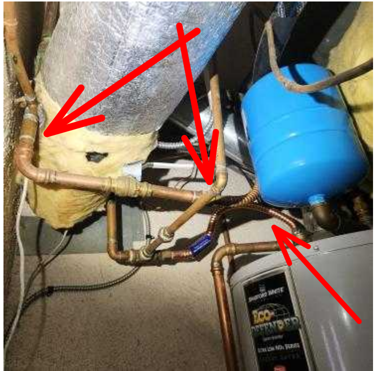
Missing insulation on supply/flow pipes to water heater-NTBS
