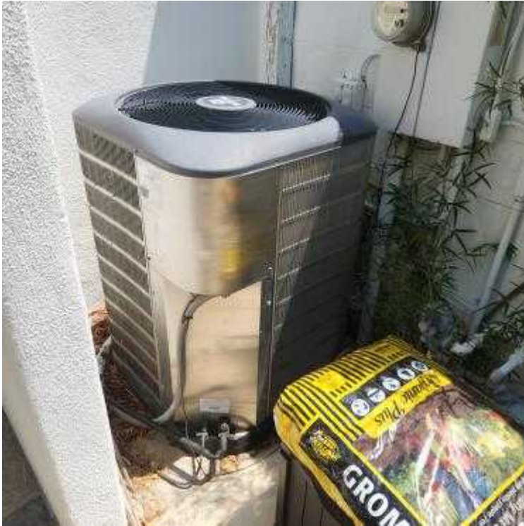
AC Condenser operated properly (5 ton 2011 model located on west side of house)
