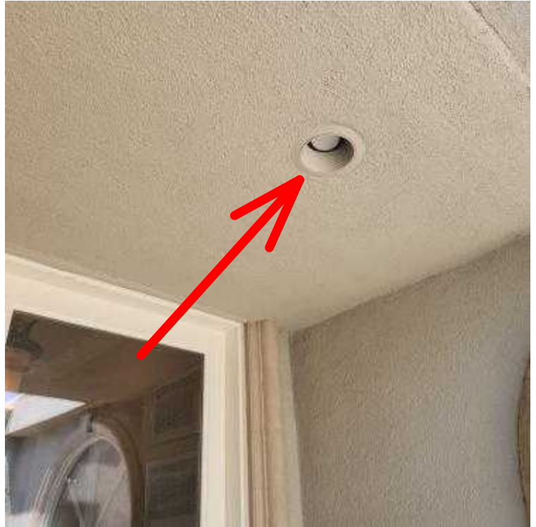
Inoperative fixture/bulb on north patio ceiling
