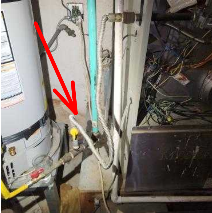
Missing sediment trap on gas supply pipe to heater-NTBS
