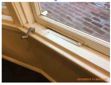
239: - One or more of the window lock were not latching/defective/missing. Suggestion: We recommend correcting the condition noted for security reasons. Location: kitchen, living room,
