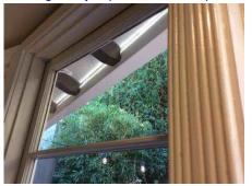
237: - The counter balance mechanism on the window(s) in the I[] were damaged and non functional. RECOMMENDATION: Replacement of the damaged mechanism is suggested. We recommend proper repair as necessary by a qualified tradesperson.
