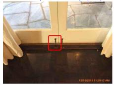
234: - The sliding glass door(s) did not operate smoothly, probably because of worn or poorly adjusted rollers. RECOMMENDATION: We recommend the track be cleaned and the rollers adjusted or replaced as needed to restore proper operation.
