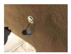
123: - One or more light(s) did not respond. This may be due to burnt/missing bulbs. RECOMMENDATION: We recommend replacement of the bulb(s). If this does not correct the condition, further evaluation and correction by a qualified electrical contractor is advised..
