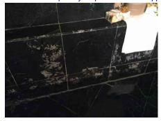
205: - The grout/caulking was deteriorated or missing in a number of areas in the tub enclosure. Suggestion: We recommend correcting this condition to prevent moisture intrusion into concealed spaces.
