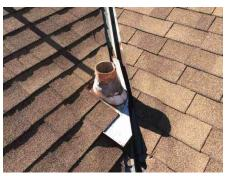
65: - There was debris on the roof. RECOMMENDATION: We recommend the debris be removed and the roof be inspected regularly.
