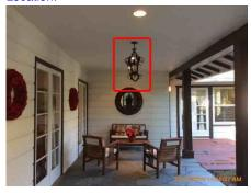
124: - One or more of the exterior light fixtures is loose from the wall and does not consist of a weather tight seal/gasket to prevent moisture penetration and deterioration. Recommend securing and sealing as necessary to prevent damage.
