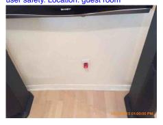
120: - Receptacles were found to have a loose/unsecured connection to the box or loose blades inside the receptacle. This is conducive to wires arcing and overheating, creating a potential fire hazard. Repair is recommended. We recommend evaluation of all receptacles and repair as necessary by a qualified electrician.
