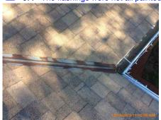
**68:** - There is evidence of corrosion of the visible flashings/vent covers. This condition does not appear to compromise their serviceability at this time. Routine maintenance should include the cleaning, sealing and spot painting of all exposed metal flashing on the roof.
