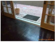
235: - There were no visible safety glass markings on the glass panes in one or more of the doors. This was not originally required but is by today's standards. RECOMMENDATION:As a safety upgrade, we recommend the glass be changed to tempered glass. Location:
