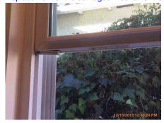
238: - Several window crank handles were stripped or missing. This condition does not allow operation of the windows. Suggestion: We recommend correcting the condition noted.
