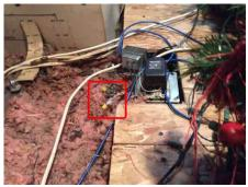
126: - Electrical cables/ wires are missing/damaged strain relief clamps where the wires enter the junction boxes. This condition allows the potential for mechanical damage to the cable and indicates non professional installation. RECOMMENDATION: We recommend correction by a qualified electrical contractor
