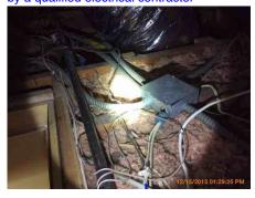
127: - The exposed wiring within six feet of the attic access opening was not protected from damage. This condition is non conforming to industry standards. RECOMMENDATION: We recommend that the wiring in this area be protected from damage for safety reasons.
