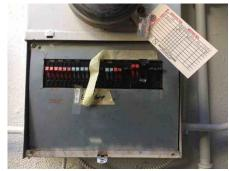
116: - The main panel is manufactured by Zinsco. Panels of this type have been known to present latent hazards by malfunctioning under certain conditions resulting in jammed circuit breakers. The breakers may not trip (disconnect) under imposed load conditions.
