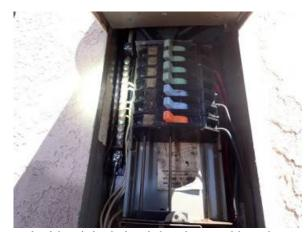
Marginal - Old panel with original circuit breakers and buss bar noted. The expected service life of a circuit breaker/ bus bar is 40-50 years. These breakers/ bus bar appear to have reached or exceeded this time frame. No damage, melting or scorching was noted at this time. However, old, outdated breakers may not perform in a reliable manner. Recommend further evaluation by a licensed electrician. Marginal - The main electrical service appeared to be outdated and undersized by
