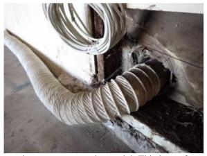
**Safety** - The flex vent is not an approved material. This is a safety concern. Corrections are needed for safety.
