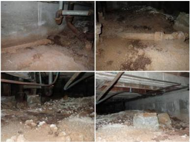
**Further Evaluation** - Moist soil conditions were present. The source of the moisture was not determined. This is usually an indication that drainage around the foundation needs to be corrected/improved but this also may be from lwaking cast iron pipes. It is important to take action in order to prevent damage to the foundation.
