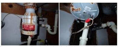
**Safety** - There are open splices in the electrical wiring to the disposal. This is a potential shock hazard. Repair is needed.
