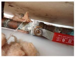
**Repair**- Corrosion was noted at the shutoff valve. Recommend further evaluation or replacement.
