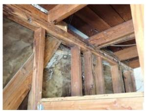
**Advisory** - Water stains were noted on the underside of the roof sheathing or framing. We suspect that the stains occurred prior to the installation of the current roof covering, however, you may wish to have a roofing contractor investigate the condition.
