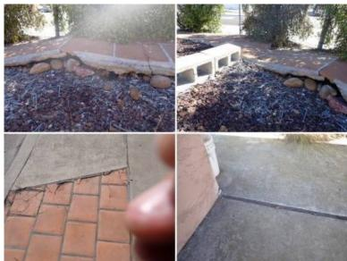
Marginal - Raised/Settled surface was noted. Repairs are recommended. Marginal - Large and/or excessive crack(s) were present.
