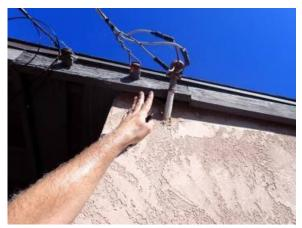
**Safety** - The overhead main service wires lacked adequate clearance. Service lines were less than 10' over walkway (accessible to pedestrians). We recommend installing a service pole and raising the service wires to the correct height for safety.
