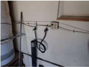
**Upgrade** - Standard rubber hoses are present, which should be replaced every 5 years to help prevent against failure. We recommend replacing with woven metal hoses for better performance/ less maintenance.
