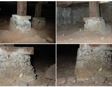
**Further Evaluation** - Deterioration was noted to some of the concrete piers. This condition is typically caused by excessive moisture is reaching the sub-area. It is important to take action in order to stop further damage to the foundation. Corrective action may include improving site drainage, as well as replacing damaged piers. Further evaluation and corrections as needed are recommended by a qualified foundation contractor.
