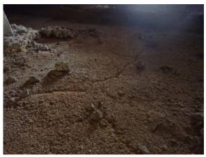
**Advisory** - Soils appeared to be clayey. Movement of underlying soils may occur with excessive moisture that could damage exterior flatwork and adversely affect the foundation. Drainage controls and restricting irrigation are advisable.
