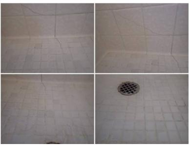
**Repair** - Tile(s) are cracked / damaged. Cracks may allow moisture into the wall causing hidden damage and the edges can be sharp. Repair / replacement is recommended by a tile contractor.
