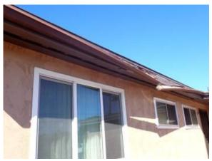
**Repair** - Moisture damage was observed. See Pest Inspection Report for damage to exterior wood members or have one performed.
