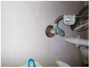
**Upgrade** - Some newer or replacement local shutoff valves and/or plumbing connections were installed serving the sinks and/or toilets. Remaining components were old/original, beyond their expected service life. These components have a 15-20 year life expectancy and are prone to failure as they age. Recommend replacing old components as an upgrade to the system.
