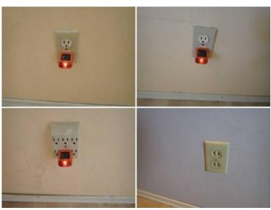
**Repair** - 3 hole grounded outlets were installed at many locations, even though no grounding wire was present throughout most of the electrical system. The use of 3 hole grounded type outlets gives the false impression of a grounded circuit. Older style 2 slot outlets are still available and should be installed. Alternatively, GFCI protection may be installed for ungrounded outlets.
