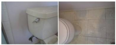
Maintenance - The toilet was loose at the floor. Recommend pulling the toilet, checking for damage, and then installing a new wax ring and caulking around the base of the toilet for added stability.
