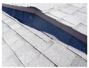
**Repair** - Metal flashing was not visible and appears to be missing at roof to wall transitions. Metal flashing is a component of the roofing system that would ordinarily be installed at this location to prevent water infiltration. This installation requires more maintenance than flashing to prevent leaking. We recommend installing metal flashing.
