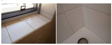
**Repair** - Tile(s) are cracked / damaged at the sill. Cracks may allow moisture into the wall causing hidden damage and the edges can be sharp. Repair / replacement is recommended by a tile contractor.
