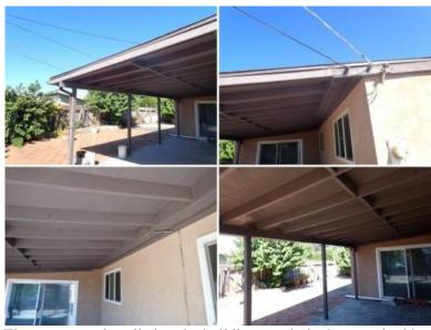
**Repair** - The rear cover is nailed to the building, not bolted as required by today's standards. This type of installation does not last as well as a bolted system and may fail in the event of seismic movement or strong winds.
