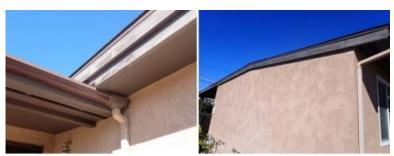
Maintenance - Gaps were noted. Gaps in exterior siding or trim should be sealed/protected to help prevent water infiltration and moisture damage.
