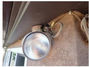
**Safety** - Open splices were noted. Wire connections are exposed, and consequently, are a shock and fire hazard. Correction is needed to contain spliced wires/connections inside a sealed junction box.
