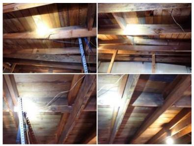
**Further Evaluation** - Split/damaged roof framing was observed. Recommend further evaluation and repair by a qualified framing contractor/ engineer at this time. **Advisory** - A storage loft was added in the garage. The storage loft relied on the existing roof framing for support. The roof framing was not designed to support additional storage loads. Consequently, only very light loads should be stored unless additional structural modifications are made.
