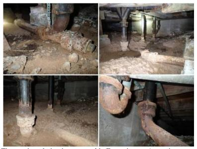
**Repair** - The cast iron drain pipes were old. Excessive rust/corrosion was present. Ongoing repairs should be anticipated as this older system continues to age. Replacing the entire system will eventually need to be undertaken. We recommend further evaluation of the cast Iron system and needed repairs made at this time by a
