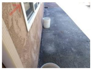
**Repair**- Replacement windows were not caulked around the top and sides of the window frame at the enclosed patio addition. Caulking is needed to prevent moisture intrusion.
