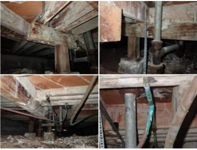
**Further Evaluation** - Water stains noted on framing or sheathing. A licensed pest inspector should evaluate this condition for possible moisture damage. Stains are an indication of a past or present leak, which should also be evaluated further.
