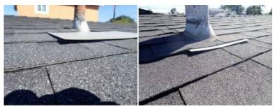
**Maintenance** - Flashing hoods/jacks had lifted. Gaps were present that can allow wind blown rain to infiltrate. Correction recommended.
