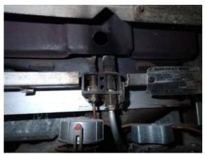
**Safety** - There are burn marks and/or rust outside of the burn chamber. This may be from combustion gases spilling out. **This should be considered a serious safety** hazard and needs further evaluation / correction.
