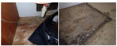
**Repair** - Moisture damage found under the sink. We recommend correcting the source of the moisture as well as replacing any damaged materials. Additionally past stains/ damage noted in the fridge zone that should be repaired/replaced.
