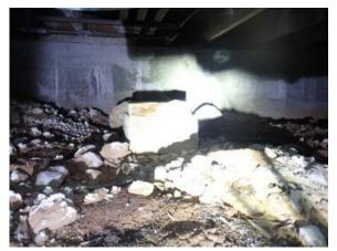
**Further Evaluation** - One pier appears to have been removed. We do not know the reason for this condition and if this pier was needed. Further evaluation and corrections as needed are recommended by a qualified foundation contractor.
