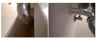
**Repair** - Deterioration/Corrosion noted to the drain line and/or wet trap under the sink. Replacement recommended.
