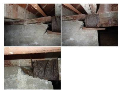
**Further Evaluation** - Lifting or gaps under the wood plate line were noted. Additionally a beam end is being supported by a sloped/ uneven section of wall rather than a horizontal surface of the appropriate depth. Further evaluation is recommended by a framing specialist/ engineer.
