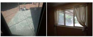
Maintenance - Glazing was dirty. Not all defective glazing may be readily apparent due to dust/dirt on the glazing. We recommend cleaning the windows and sliding doors and checking for any glazing issues. Seals on double pane glazing are normally covered under the manufacturer's warranty for a minimum period of 5 year and often longer. Recommend checking the warranty period and to see if the warranty is transferable.
