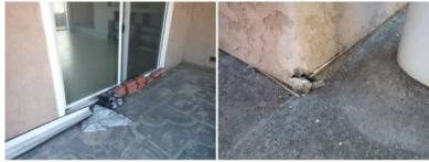
Marginal - The finished grade level of exterior flatwork was too high against the building at the patio slab addition. Ideally, the exterior flatwork should be held at least 2" below the bottom edge of the siding to help protect the siding and structure against moisture damage and termite infestation.
