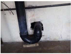
**Safety** - Hole(s) were noted in the drywall between the garage and the crawlspace/ floor framing. This interrupts the integrity of the fire separation wall. All holes should be filled with an approved material.
