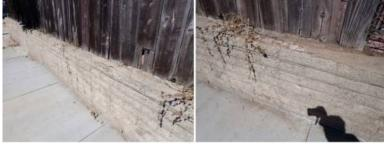
Marginal - Surface deterioration and water stains noted to the wall. This is usually an indication that the waterproofing and/or drainage system behind the wall is damaged or insufficient.
