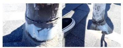
**Maintenance** - Sealant around vent penetrations is cracked/deteriorated. Fresh sealant is needed at this time to prevent leakage.
