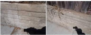
Maintenance - Moderate cracks / movement are present in the wall. Cracking of this nature is not uncommon and is an indication of modest movement/settlement in underlying soils. Generally, repair or sealing of these cracks is recommended to prevent moisture infiltration, which can cause further damage.
