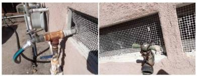
**Maintenance** - Vent screen(s) were damaged or missing. Openings were present where pests/rodents could enter.
