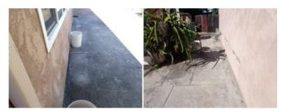
Marginal - Paved surfaces directed surface runoff toward the foundation or were flat against the foundation. Paving abutting the structure should not be pitched so that surface runoff collects against the foundation. Corrective measures recommended.
