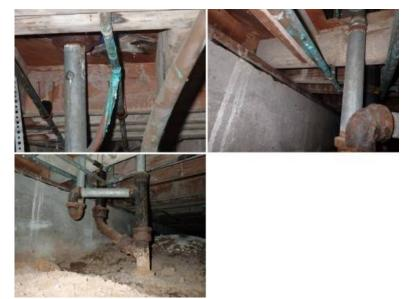
Marginal - Corrosion was noted on several sections of piping under the house. The component was showing signs of advanced aging and likely would have limited remaining life. Be aware that old corroded pipes and fittings are at a higher risk of leaking. Recommend a licensed plumbing contractor for further evaluation.
