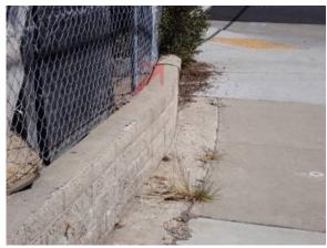
Marginal - The mortar cap or cap blocking was loose. The wall cap is in need or repair ed to prevent moisture from entering the top of the wall.
