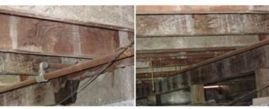
**Maintenance** - Corrosion was noted on iron gas pipe(s). Routine maintenance is needed. A rust inhibitor should be applied to prevent further deterioration.
