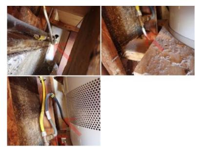
**Repair** - An old type solid brass or aluminum gas connector was noted in the garage. This ductile metal tubing can become brittle with age and susceptible to crimping and cracking. Additionally appliance connectors were being used as gas distribution (not at appliances). Repairs are recommended at this time for safety.
