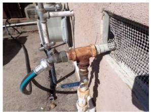
**Upgrade** - Anti-siphon device is missing at one or more locations. Installing anti-siphon devices at all hose connections will protect the potable water supply from possible cross contamination.
