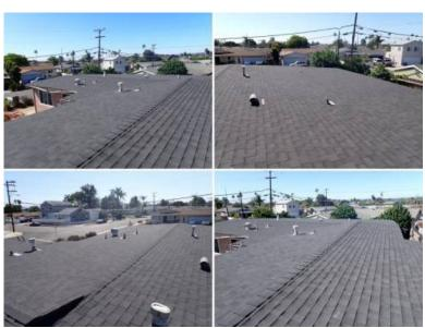
**Repair** - The roof pitch was not sufficient for the type of roof covering installed. Problems associated with this include excessive moisture retention, moisture infiltration or leaking, and limited service life. A licensed roofing contractor should be called to make further evaluation and corrections as needed.
