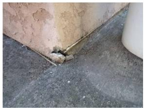
**Maintenance** - Small areas, typically at corners or bottom edge of the stucco siding, were chipped, loose or missing. Routine repairs recommended.
