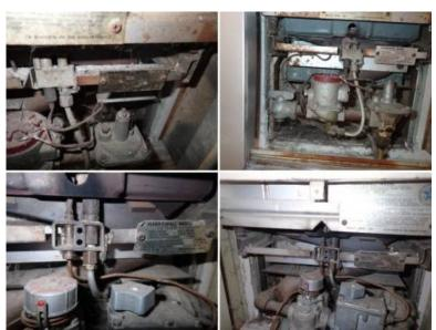
**Safety** - The wall furnace(s) did not have the safety spill sensors that are present on newer heaters. These sensors will turn off the heater if the vent does not work properly, possibly saving someone's life. Recommend up grading to a newer and safer heating system.
