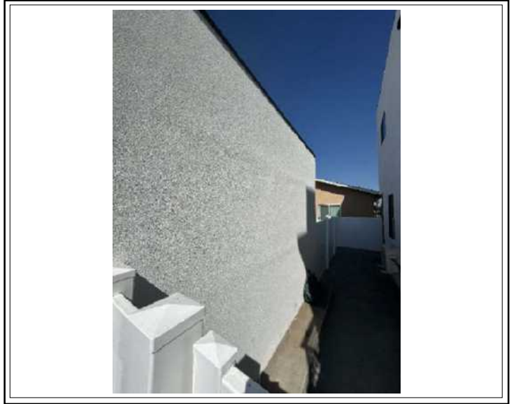
Exterior Side Unit 4128
