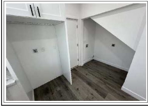
Laundry (First Floor) Unit 4130
