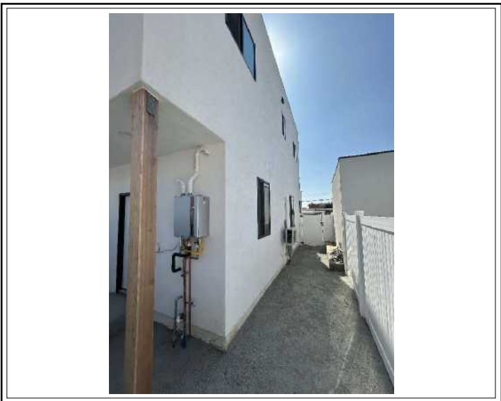
Exterior Side Unit 4130
