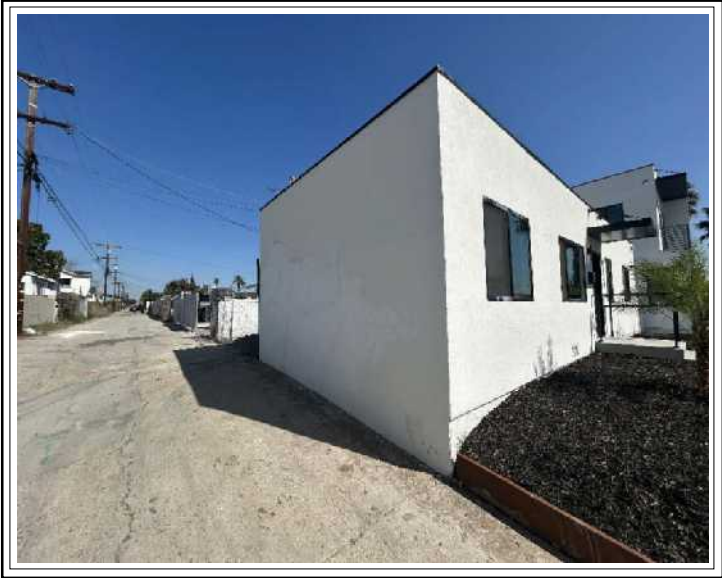
Exterior Side Unit 4128
