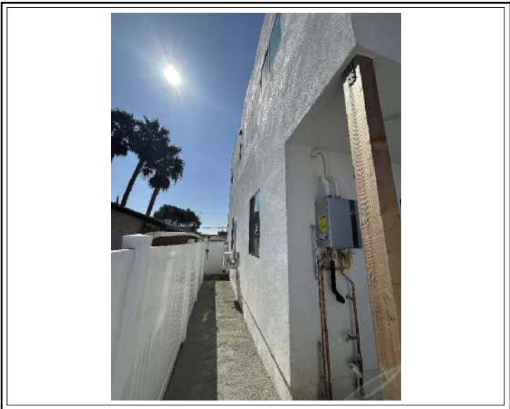
Exterior Side Unit 4132
