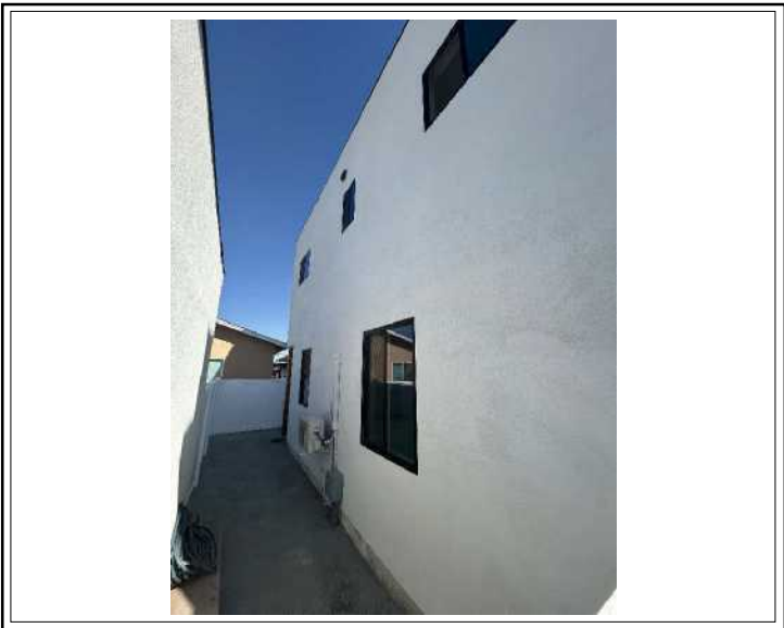
Exterior Side Unit 4130
