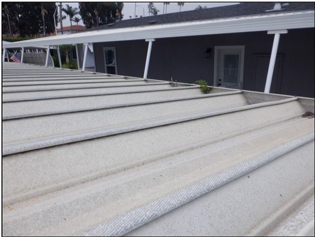
1.0 Item 17(Picture) Roof covering
