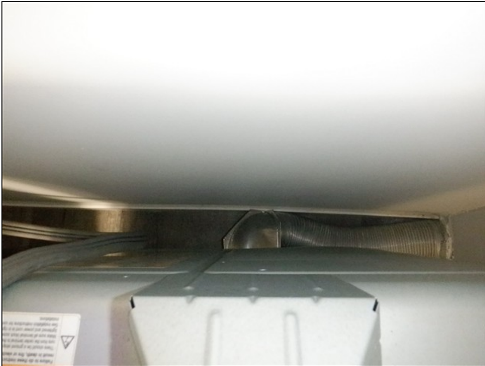
3.13 Item 6(Picture) Dryer vent
