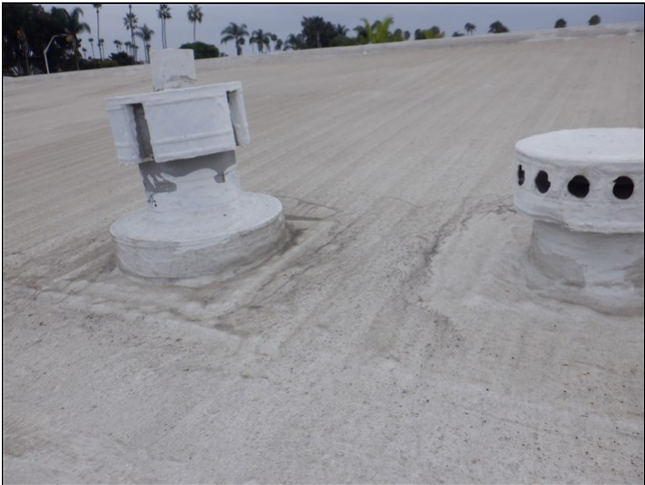
1.0 Item 6(Picture) Roof covering
