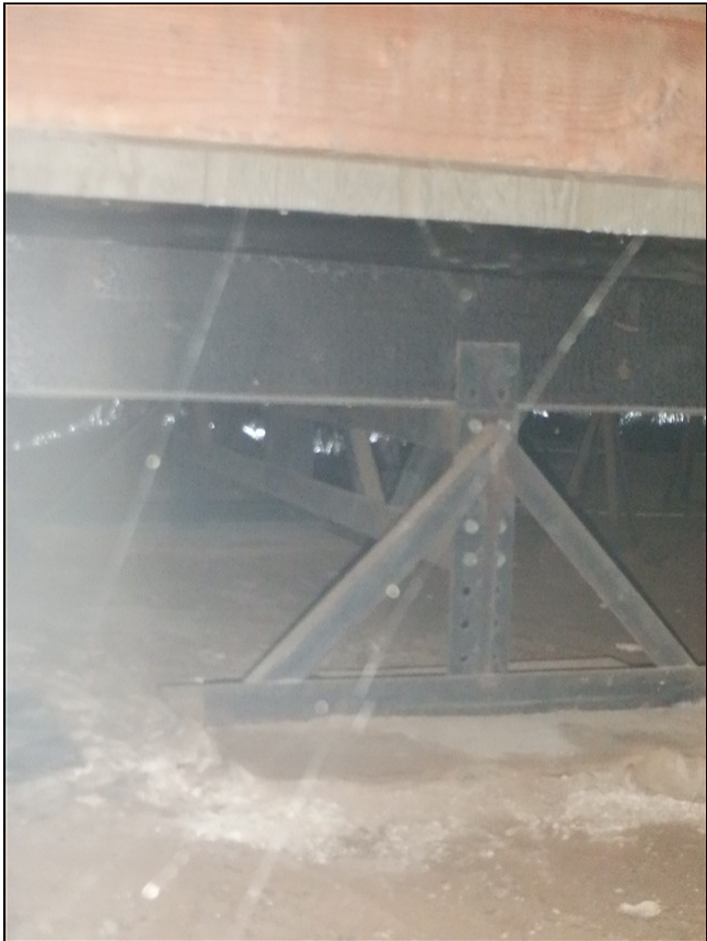
6.2 Item 3(Picture) Earthquake supports
