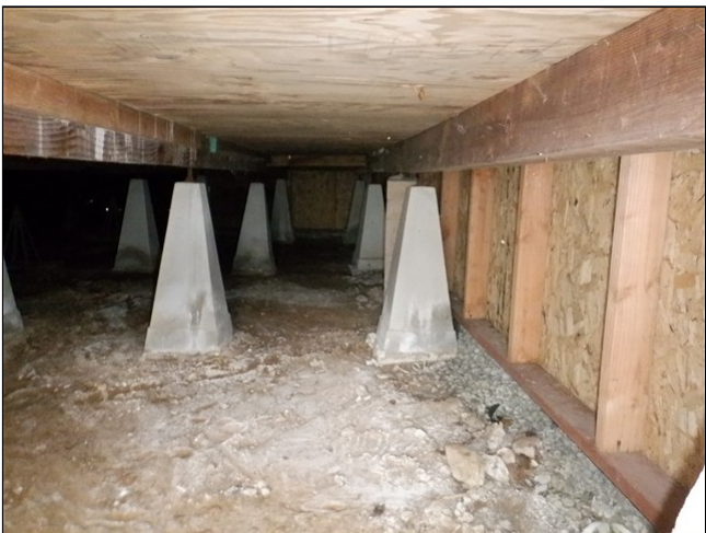
6.2 Item 2(Picture) Concrete piers under deck
