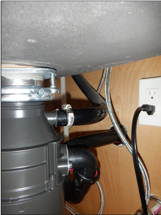
3.5 Item 1(Picture) Kitchen sink plumbing / no leaks
