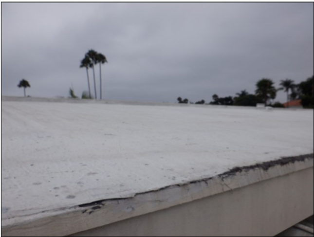
1.0 Item 14(Picture) Roof covering
