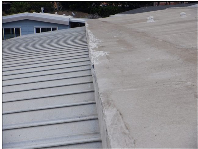
1.0 Item 3(Picture) Roof covering
