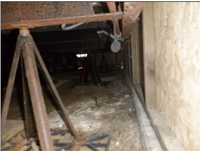
6.0 Item 2(Picture) Crawlspace
