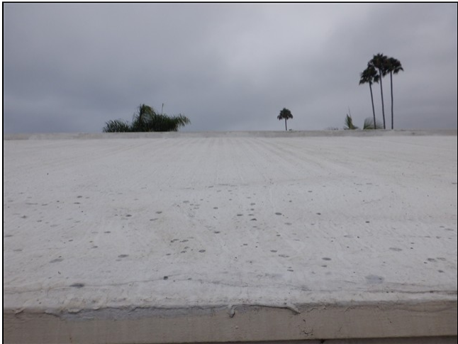
1.0 Item 15(Picture) Roof covering
