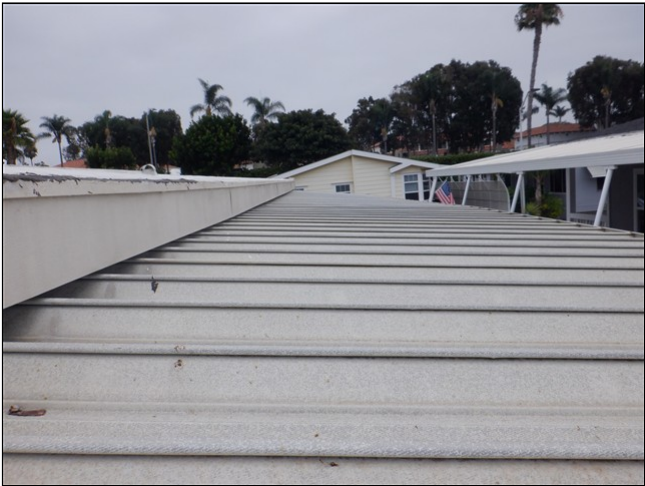
1.0 Item 12(Picture) Roof covering
