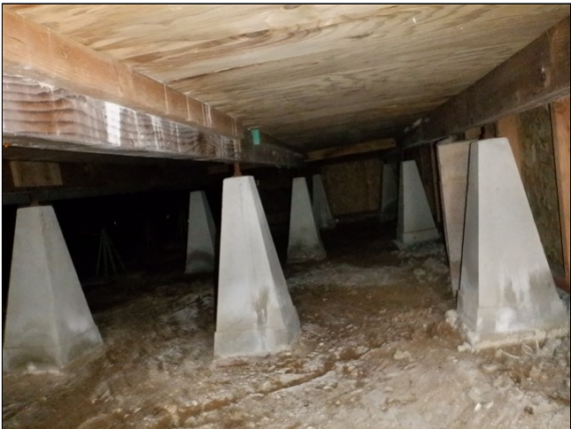
6.2 Item 6(Picture) Concrete piers
