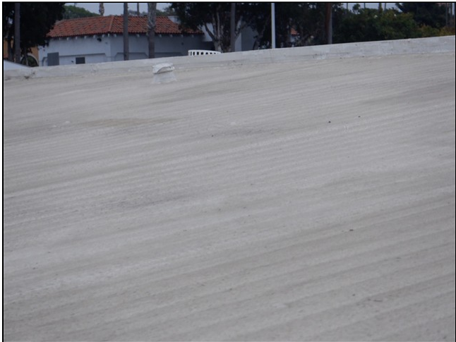
1.0 Item 5(Picture) Roof covering
