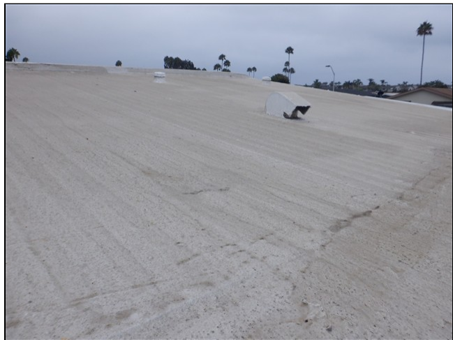
1.0 Item 1(Picture) Roof covering
