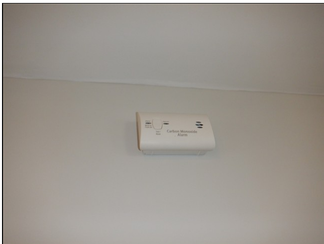
8.6 Item 1(Picture) Carbon monoxide detector
