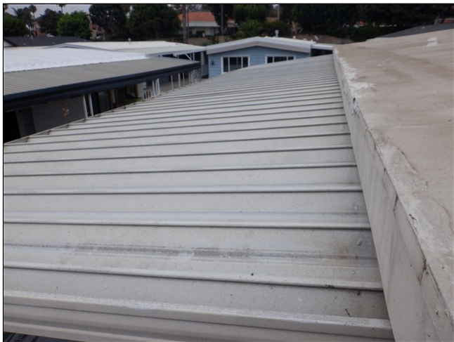
1.0 Item 2(Picture) Roof covering
