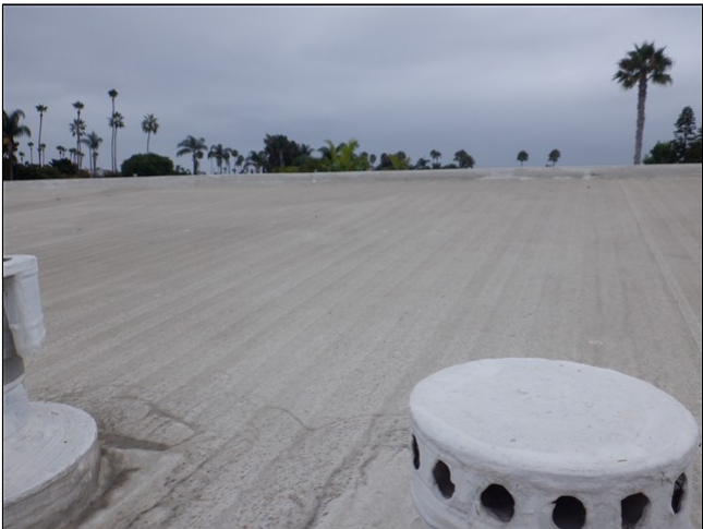
1.0 Item 8(Picture) Roof covering
