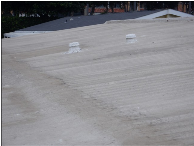
1.0 Item 4(Picture) Roof covering
