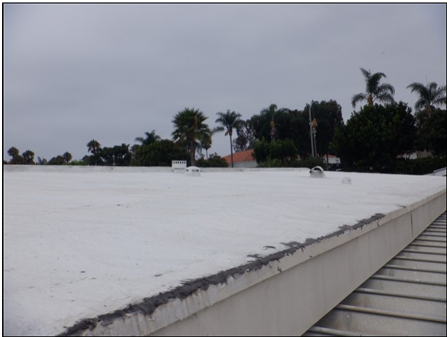
1.0 Item 13(Picture) Roof covering
