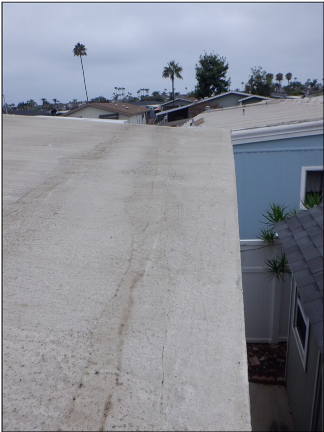
1.0 Item 7(Picture) Roof covering
