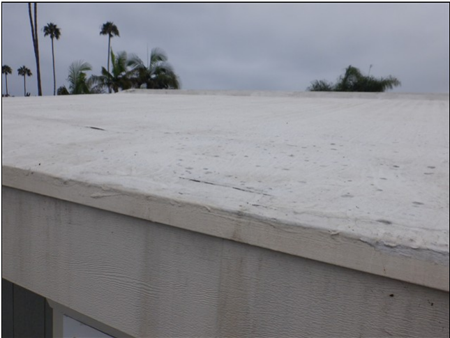
1.0 Item 16(Picture) Roof covering
